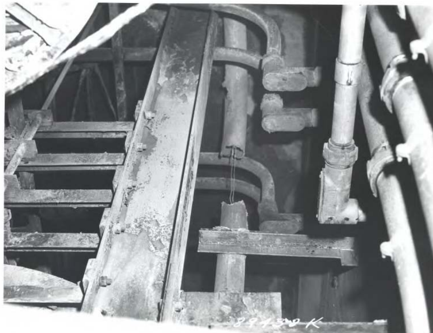
Figure A-1: Photograph of Conduit Damaged from Fire (NUREG/BR-0361)
