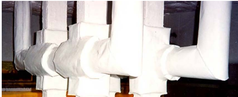
Figure 5-14. Photo of Mecatiss ERFBS (NRC Photograph)
