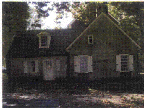
Photo 4. Stucco area (east end of house)
