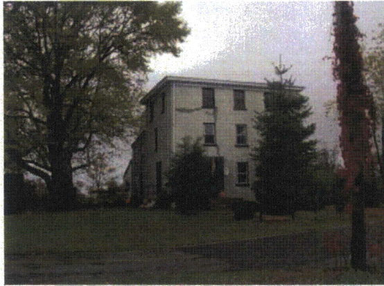
Photo 34. General view of Mason House
