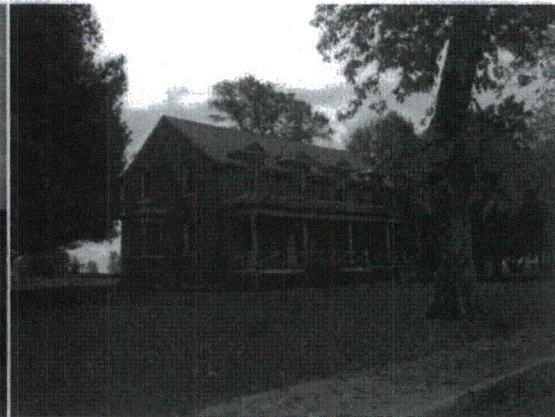
Photo 68. Bldg. north of Gov. Bacon Center
