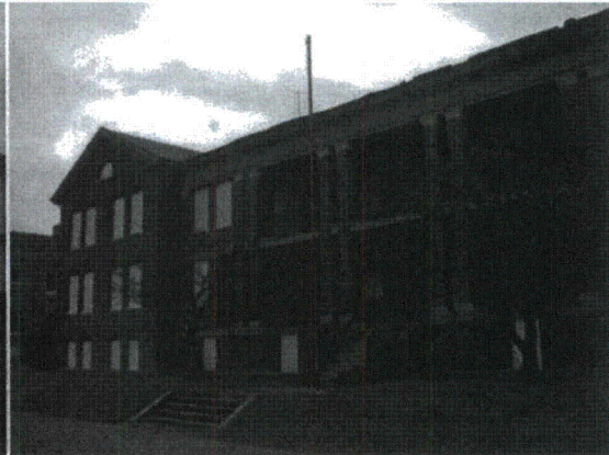
Photo 66. Building along Kent Avenue
