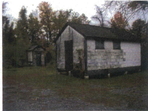
Photo 22. Tool shed and small outbuilding
