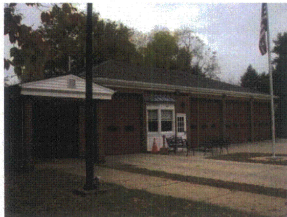
Photo 44. Modern Structure- Odessa Fire Department
