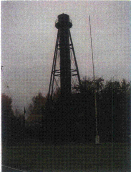
Photo 21. General view of Rear Range Light
