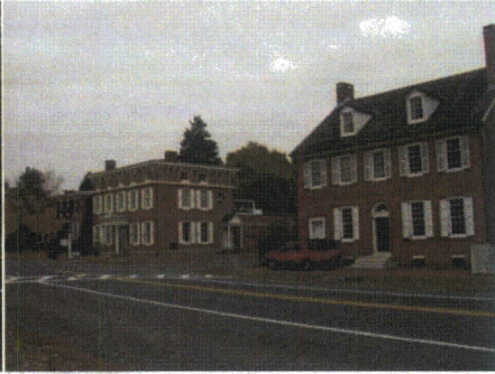
Photo 41. General View of Main Street
