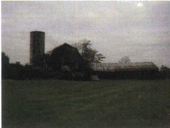
Photo 87. Outbuildings at Liston House
