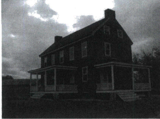
Photo 85. Gen. View of Short's Landing Hotel Complex
