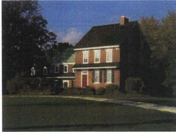
Photo 27. General View of the Benjamin Holmes House, Front
