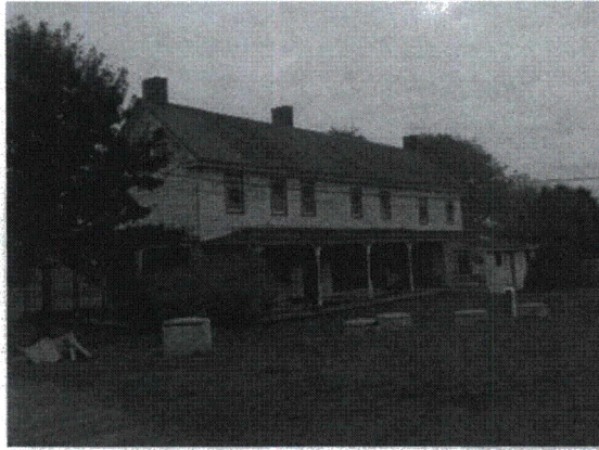
Photo 105. View of South side of Biddle House
