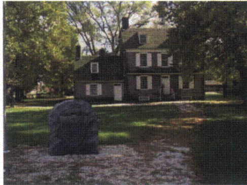
Photo 2. Hancock House, general view
