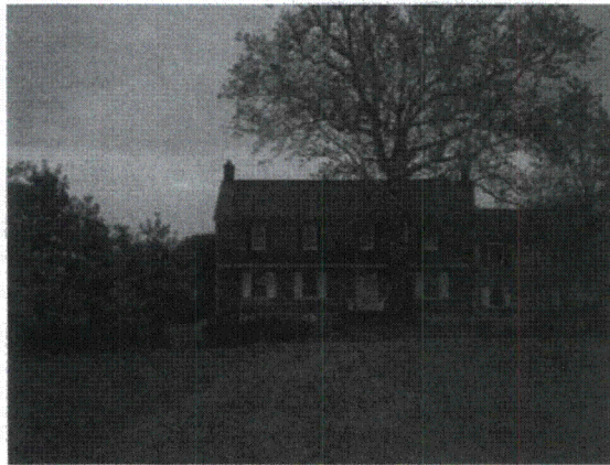
Photo 91. General View of Huguenot House
