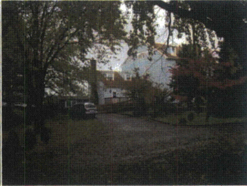
Photo 31. View of addition of South side of house
