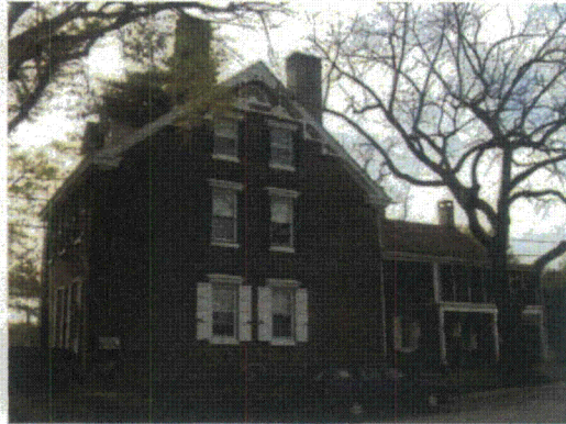
Photo 56. View of North side of Sutton House
