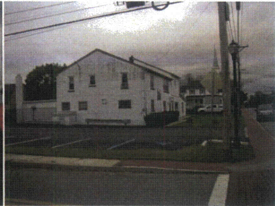
Photo 75. Commercial Building on Market Street
