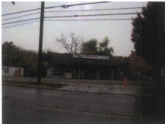
Photo 14. Modern commercial building
