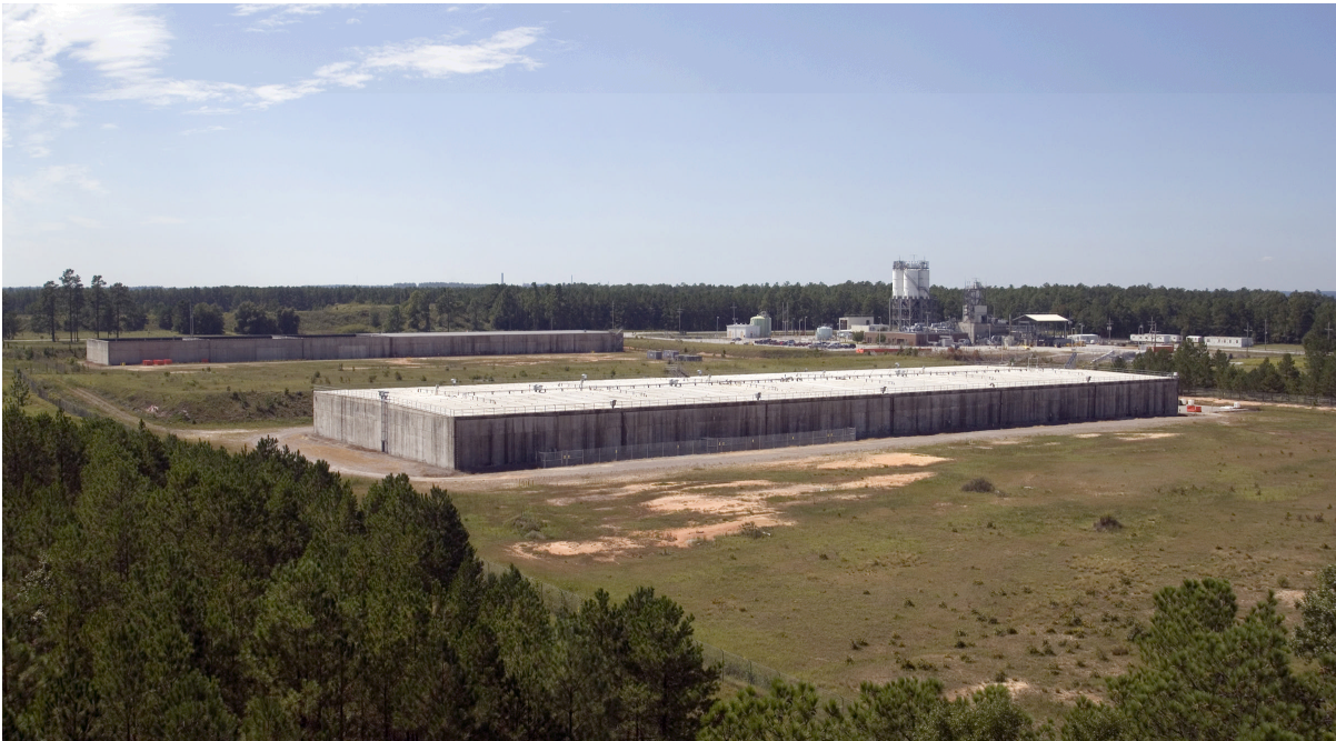
Figure 2. Aerial photograph of Z-Area showing Vault 4 (foreground), Vault 1 (background, left) and grout mixing plant and supporting infrastructure (background, right).
