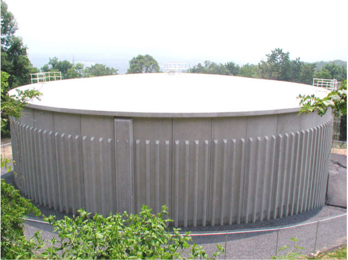
Figure 11. Photograph of a commercial reinforced concrete water storage tank ( http://www.dutchlandinc.com/product_pages/circular_5_lewistown.html , 11/17/08).
