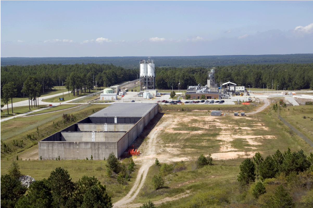
Figure 5. Aerial photograph of Vault 1 looking to the north.
