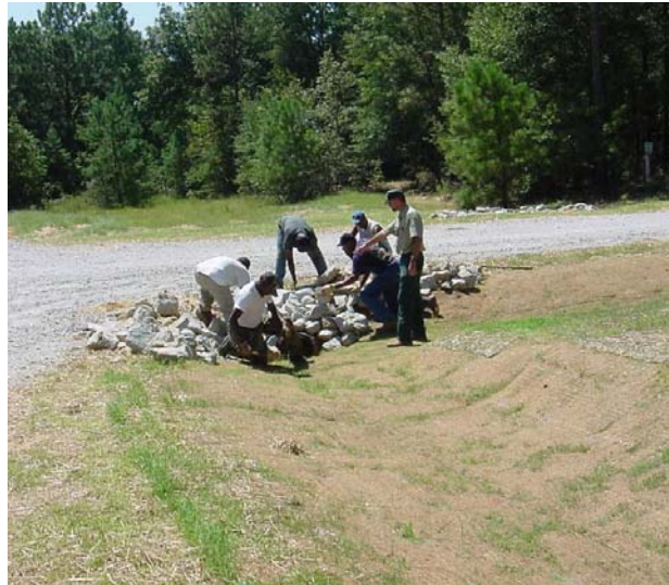
Photograph 8. Stabilization projects minimize soil movement into surface waters
