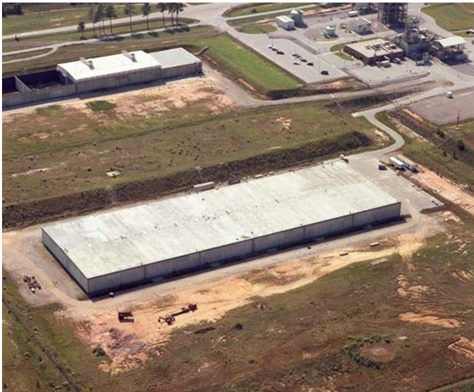
Figure 3-3. View of SDF Vault 4
