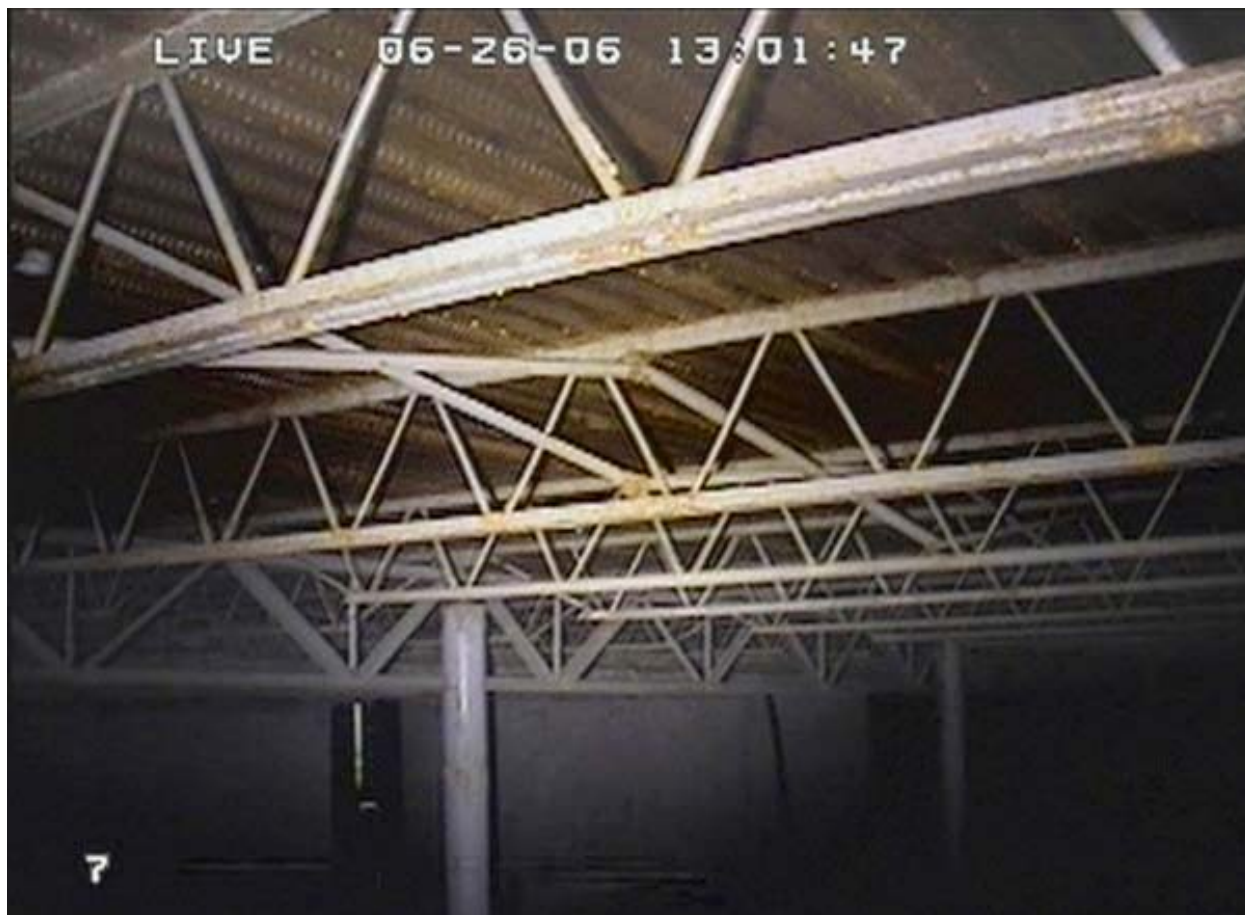
Figure 3.2-12: Interior View of Vault 4 Roof
