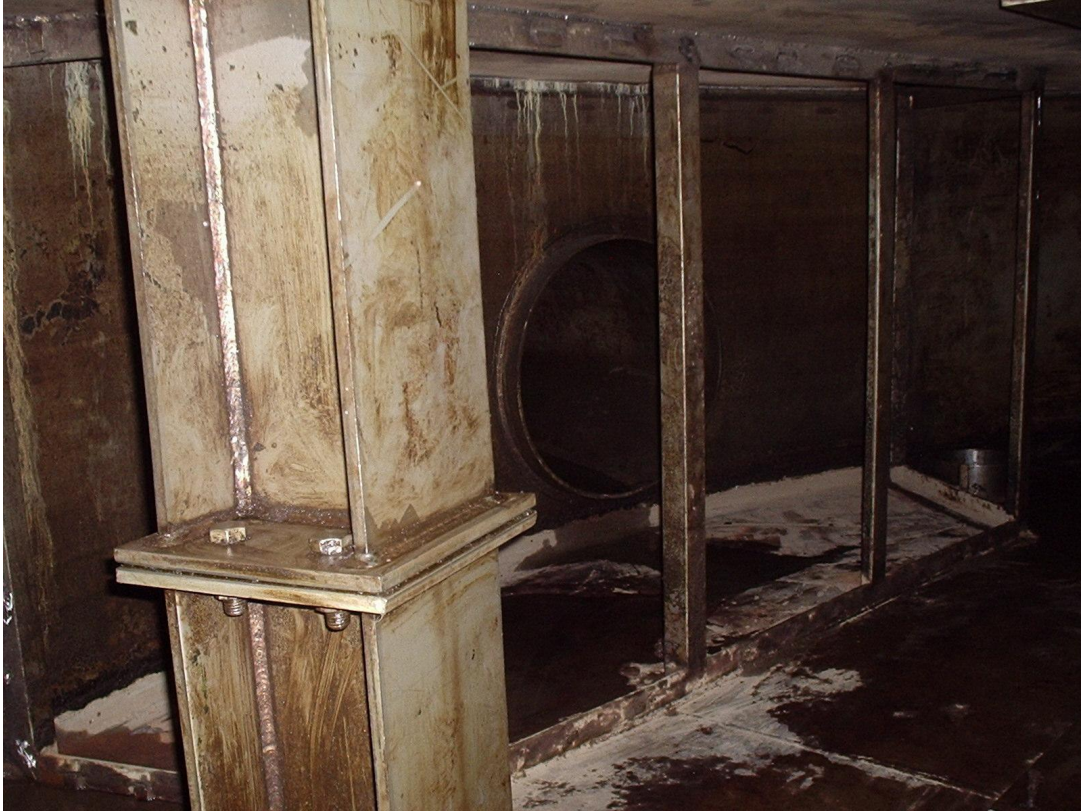
CR-PLP-2007-5055 Photo of 1 of 2 Sump Exits with Old Screen Removed White material is dried Boric Acid
