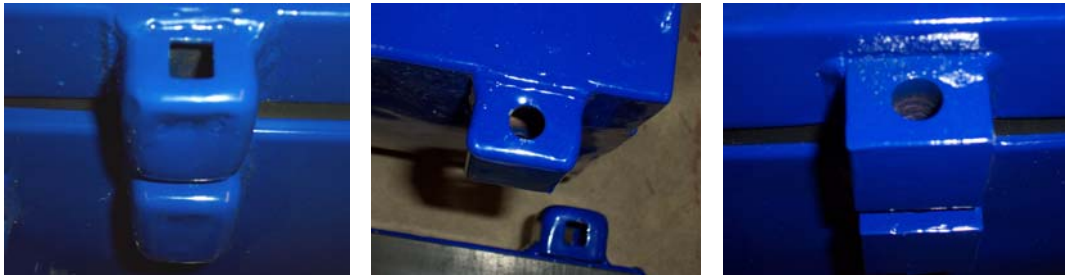
Figure 11: Bolting lug configurations
