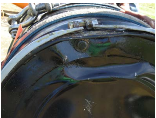
Close-up of Closure End Damage
