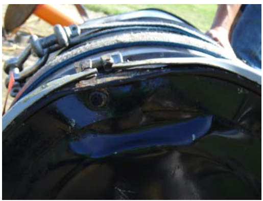
Impact Damage to Closure End
