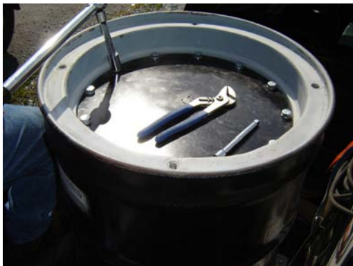
Bolted Inner Blind Flange and Top Gasket
