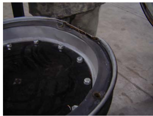
Top End Impact Area Damage
