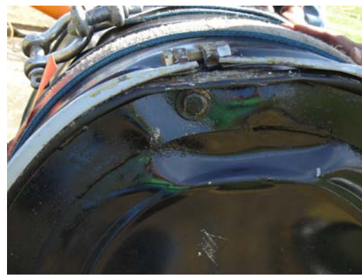
Close-up of Closure End Damage
