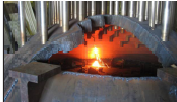
Sectioning of reactor vessel head penetrations from Washington Nuclear Power, Unit 1, a canceled plant
