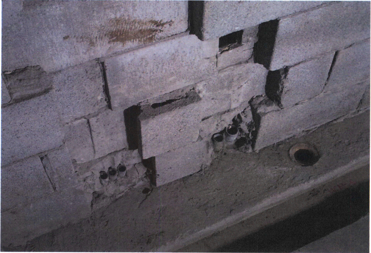
Exhibit 12, Basement Men's Room Showing Extensive Remediation (RO-3-6, Class 1)
