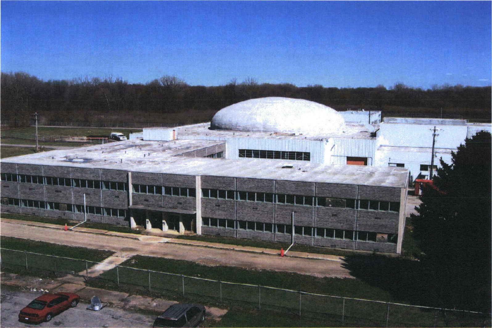
Exhibit 1, View of PBRF Showing ROLB and Reactor Building
