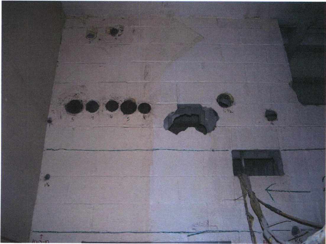
Exhibit 10, Sump Room North Wall Showing Penetrations (RO-3-10, Class 1)
