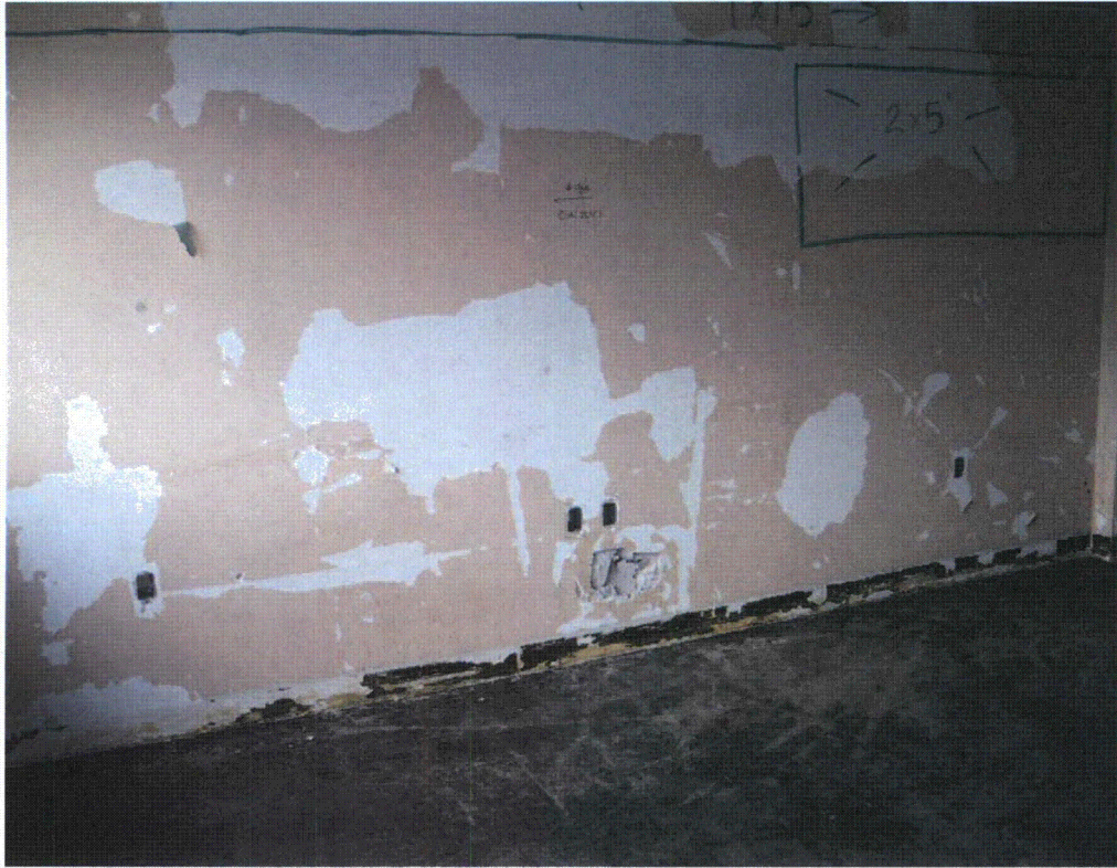
Exhibit 7, Room 109 Floor and Lower Wall (RO-1-11, Class 3)
