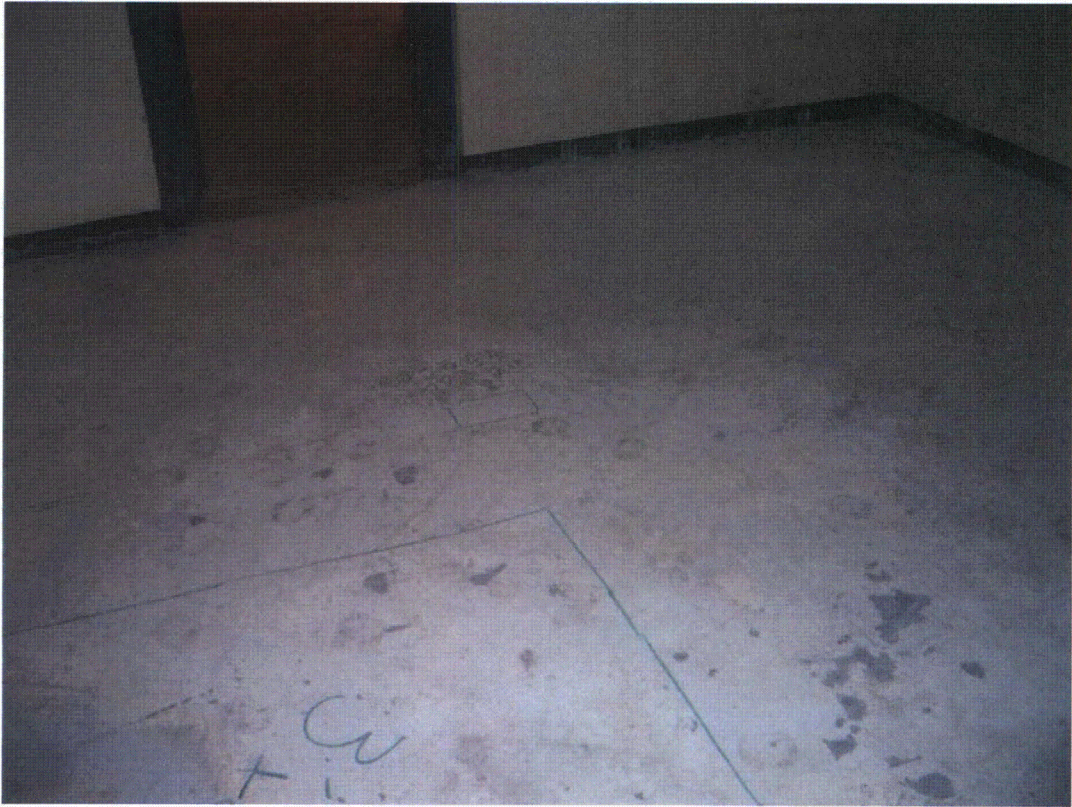
Exhibit 11, New Fuel Vault Floor and Lower Walls (RO-3-4, Class 1)
