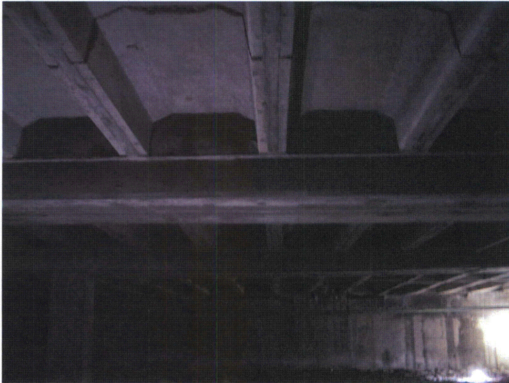
Exhibit 13, Basement Crawl Space Showing Poured Concrete Ceiling (RO-328A, Class3)
