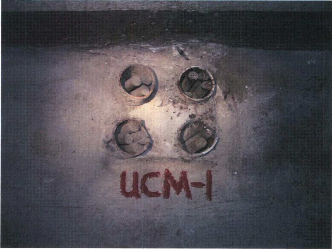
Exhibit 15, Sump Room Showing Example of Unusual Condition Measurement (UCM) Area
