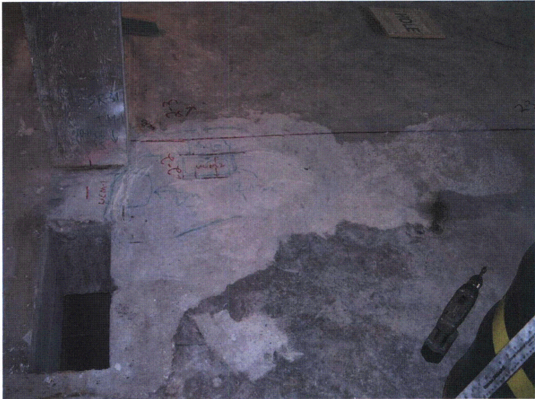
Exhibit 8, Room 209-210 Laboratory Floor Showing Remediated Area & Penetration (R0-2-2, Class 1)
