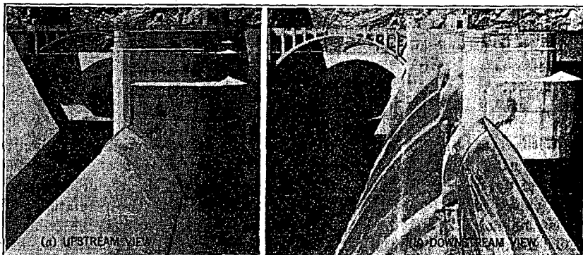
FIG. 1.—DRUM GATE, 100 FT BY 16 FT, AT HOOVER DAM (ARIZONA-NEVADA)
