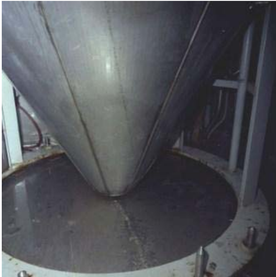
Figure 6.3-3: View of the Bottom of the 242-25H Evaporator Vessel
