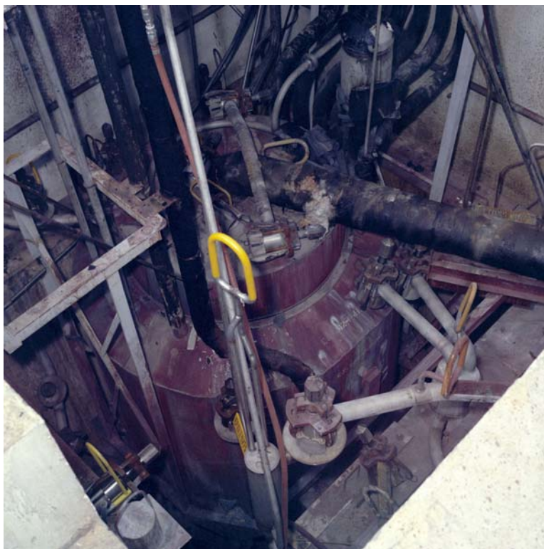
Figure 6.2-2: Top View of the 242-16H Evaporator Vessel
