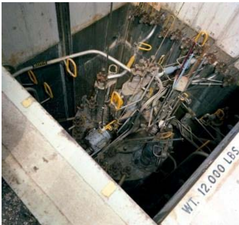
Figure 4.5-1: HTF CTS Pump Pit and Pump Tank
