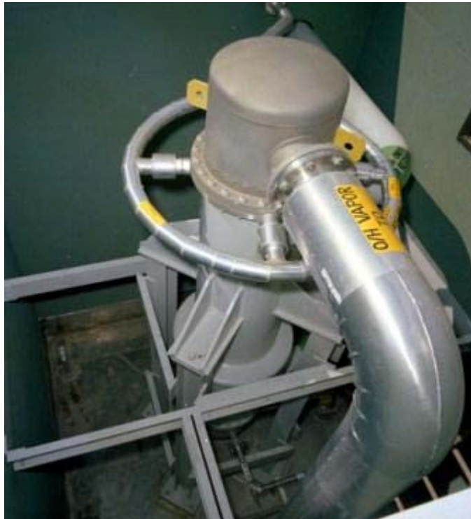
Figure 6.3-4: 242-25H Evaporator Overheads System Condenser
