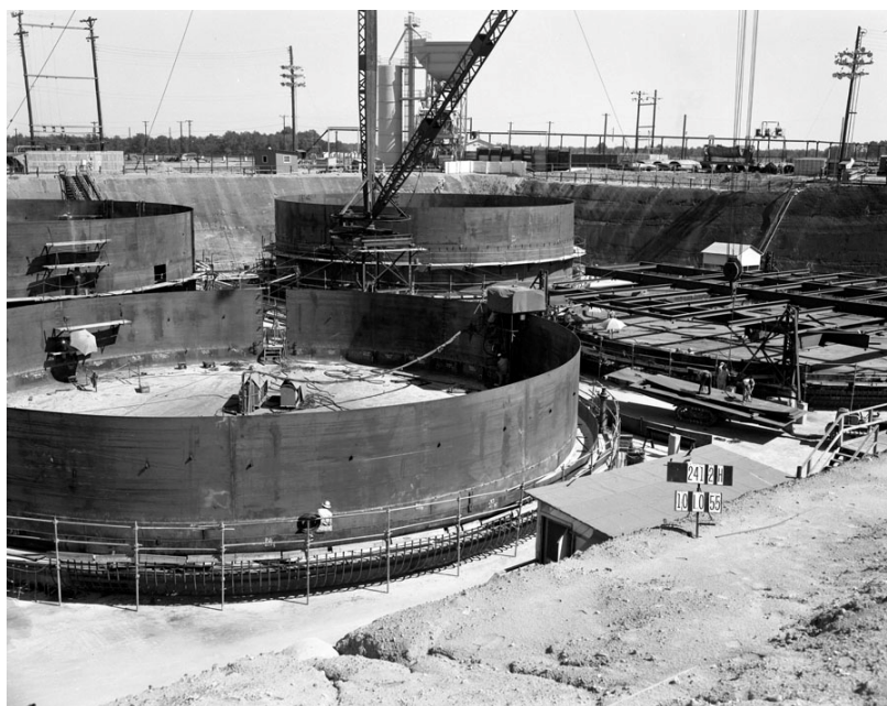
Figure 6.1-2: Type II Tank Primary and Secondary Liner Construction
