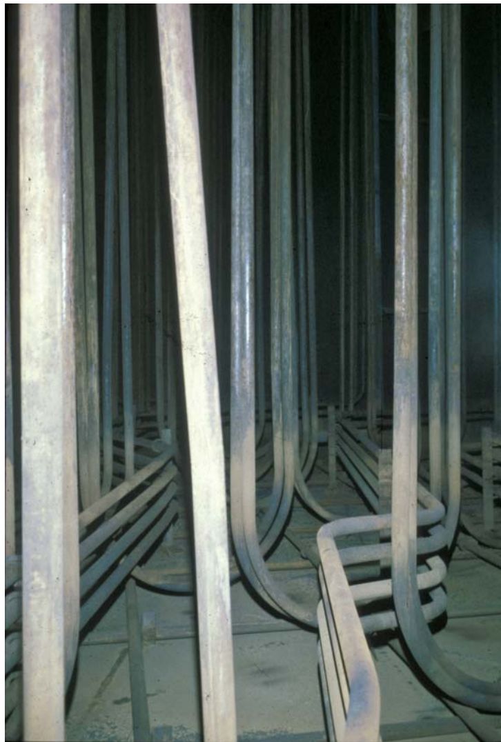
Figure 8.1-1: Type II Tank Cooling Coils
