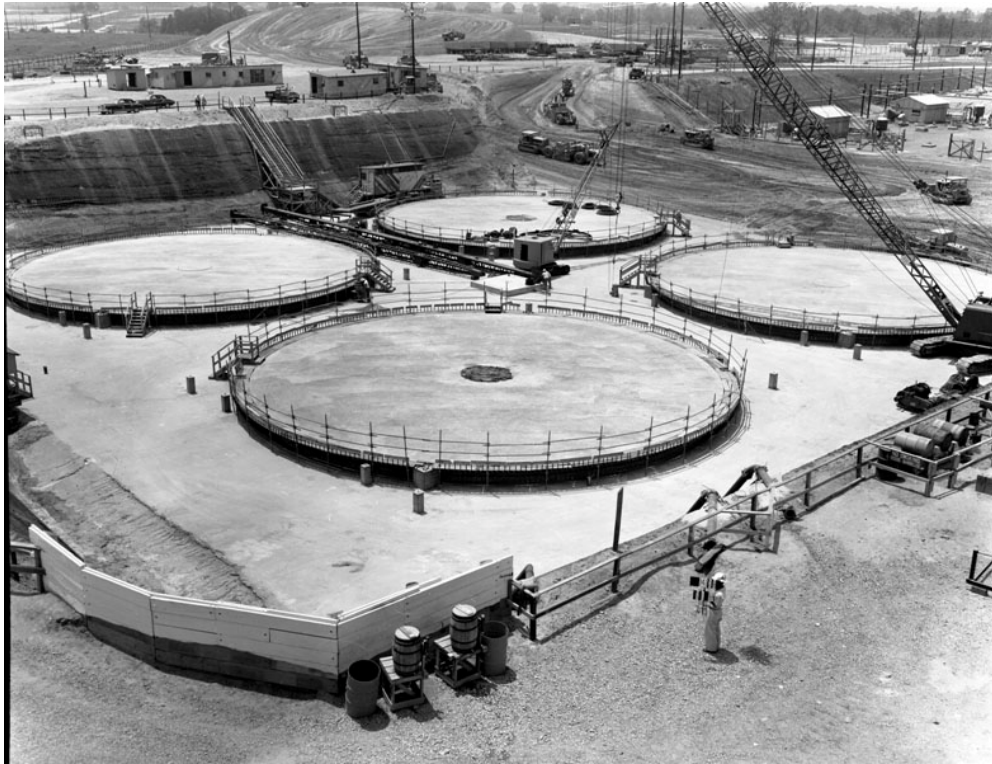
Figure 4.1-1: Type II Tank Working Slab and Basemats
