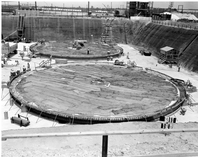
Figure 6.1-1: Installing Lower Sand Layer over Basemat
