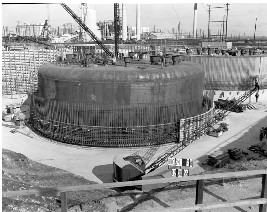
Figure 7.1-1: Early Stage of Type II Tank Vault Construction
