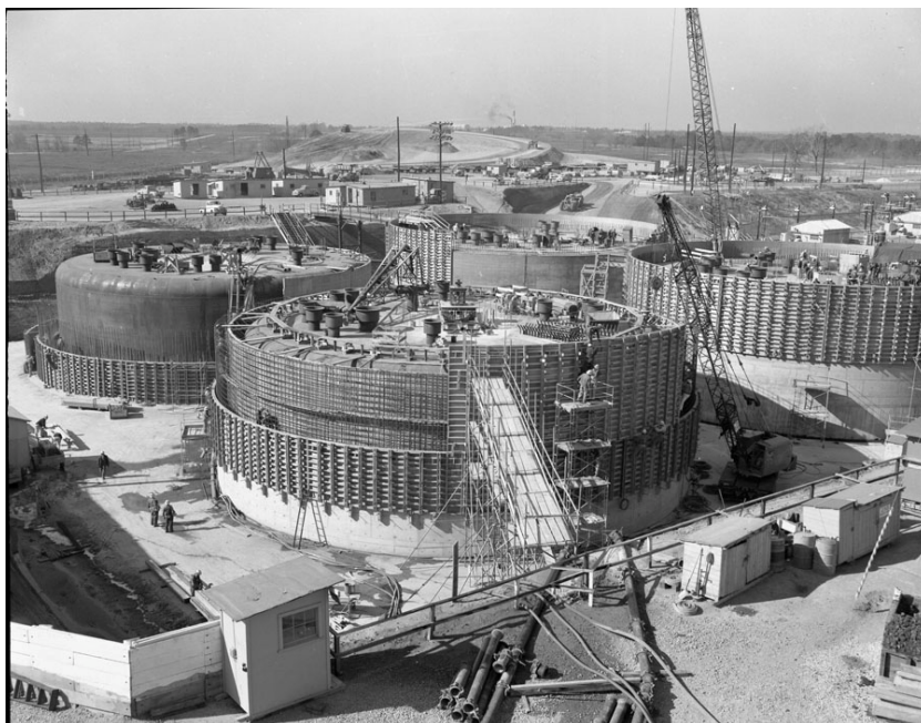
Figure 7.1-2: Later Stage of Type II Tank Vault Construction
