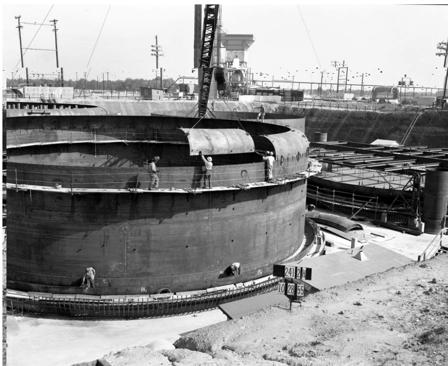
Figure 6.1-3: Type II Tank Placement of Upper Knuckle
