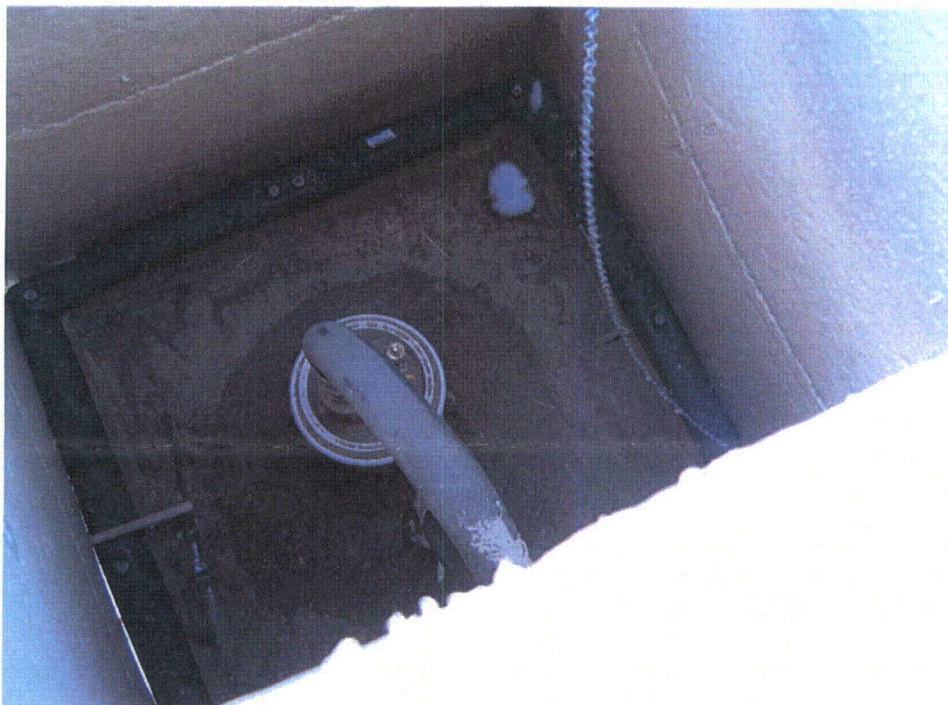
Figure 4 View of inside of well in Figure 3
