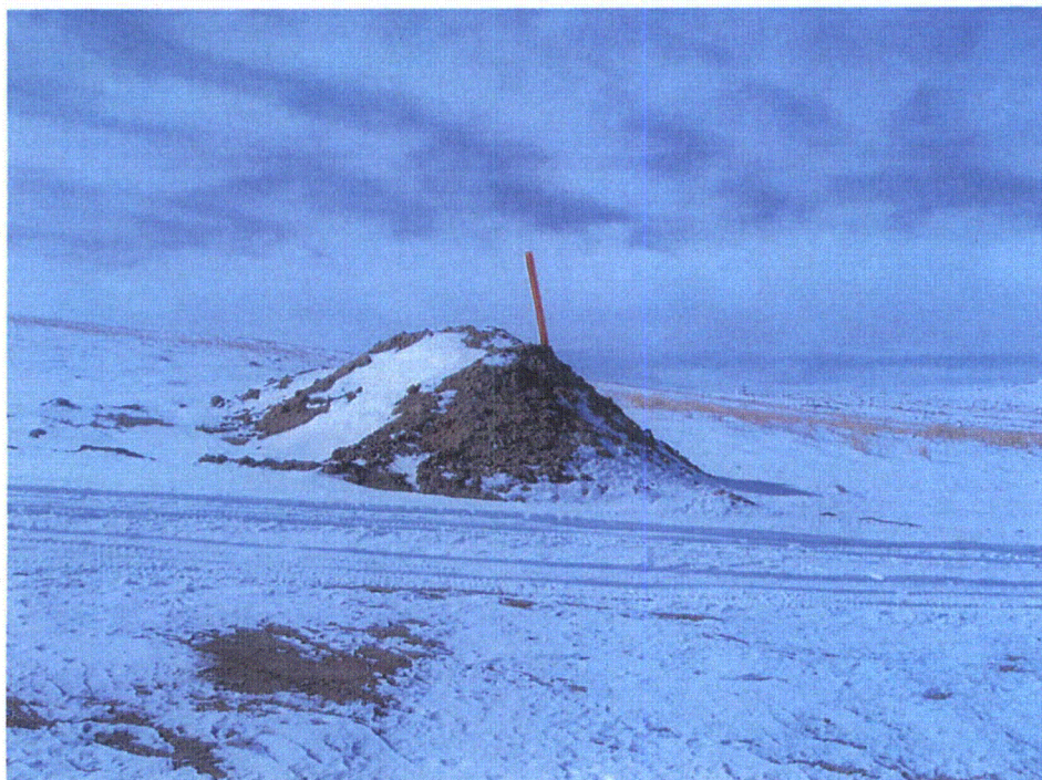
Figure 2 Topsoil stockpile with sign
