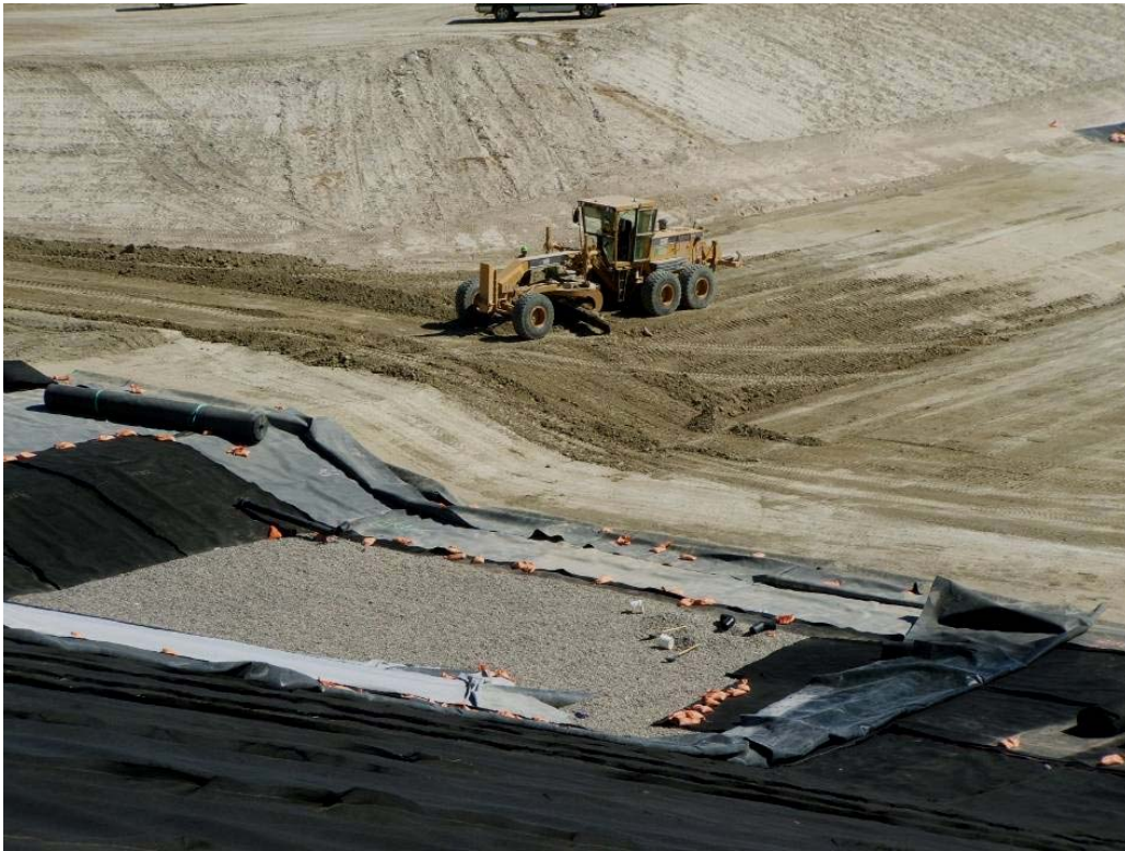
Figure 1-7 Cell 15 Liner Installation
