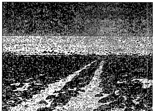
Photographs 3 and 4. Exterior of the east embankment, showing some external rilling.
