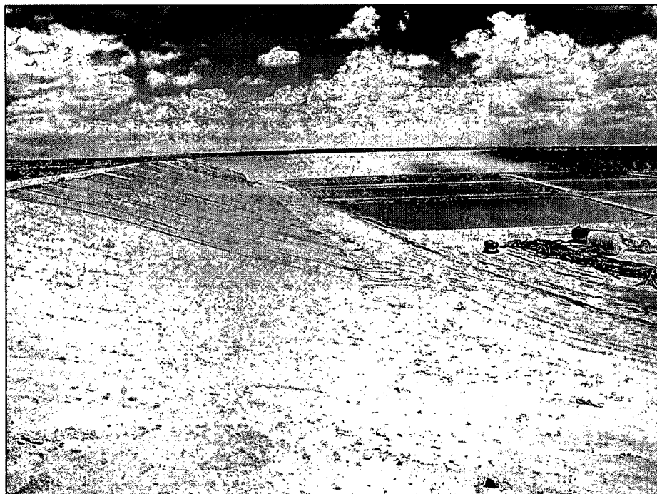
Photograph 4. West half of north embankment; functional liner between bench and crest; also note evaporation lagoons on tailings surface.
