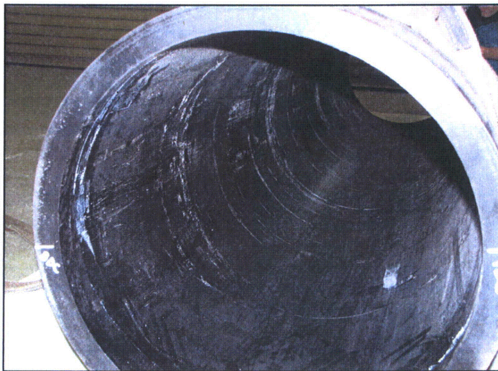
Figure 83 – NS30 #2 Body Pipe After Removal of Bottom End Cap
