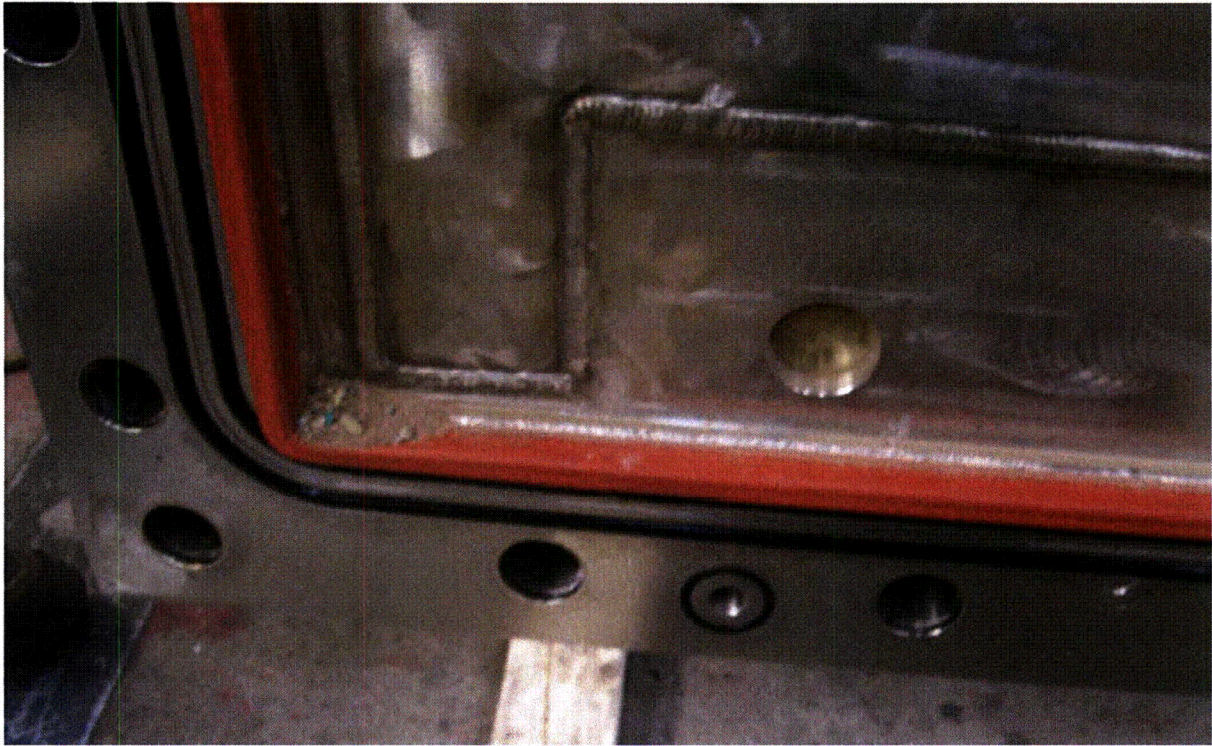
Figure 2.12.6-17 – Debris and Debris Shield (red) Upon Closure Lid Removal
