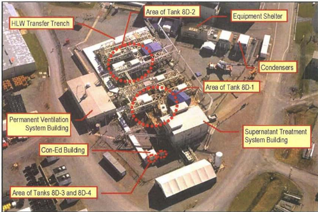
Figure C.10 WMA 3 Oblique Aerial Photograph (from Phase 1 DP, Figure 3-30)
