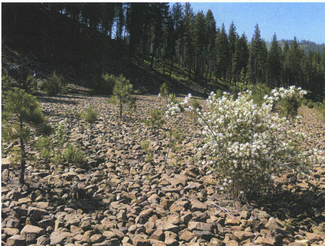
LOW 7/2009. PL-3. Vegetation on the disposal cell cover.
