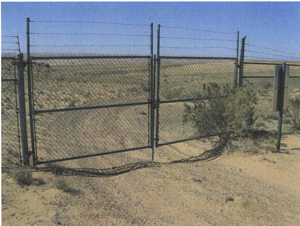
TUB 4/2009. PL-1. Gap under the vehicle gate at the southeast corner of the site.
