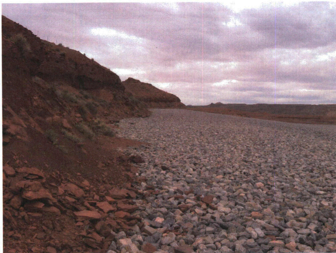
HAT 4/2009. PL-4. Erosion of rock and soil onto the riprap apron all along this section.
