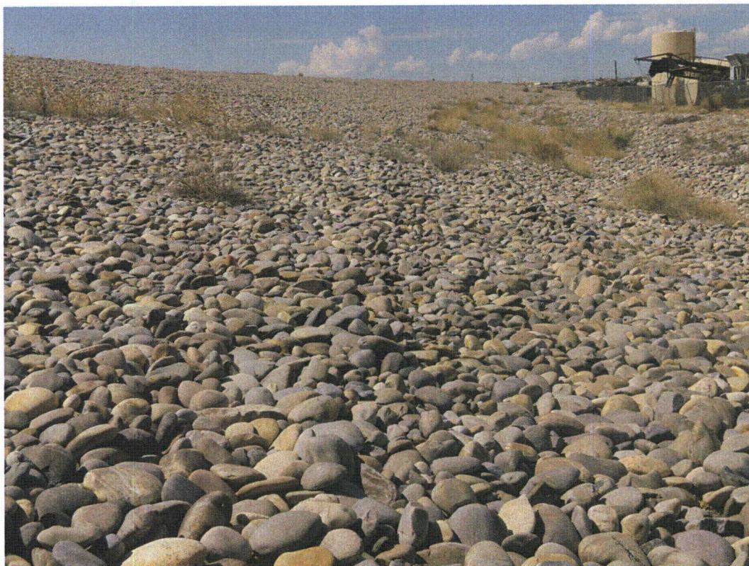
SHP 5/09. PL-3. Dead vegetation on the disposal cell slopes and drainage channel.
