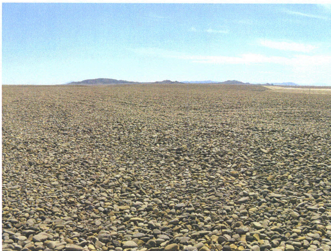
SLC 4/2009. PL-4. Slight depressions southwest of site marker SMK-2 on the disposal cell top.
