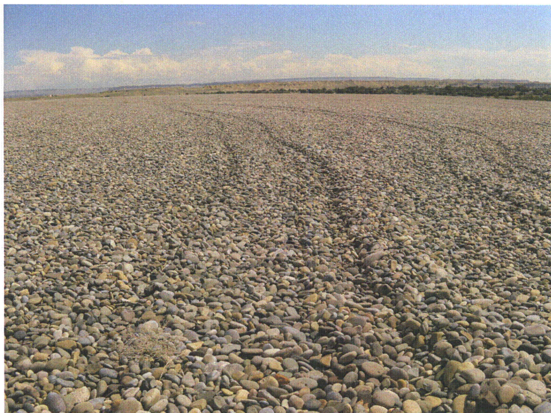
SHP 5/09. PL-2. Vehicle ruts on the surface of the disposal cell.
