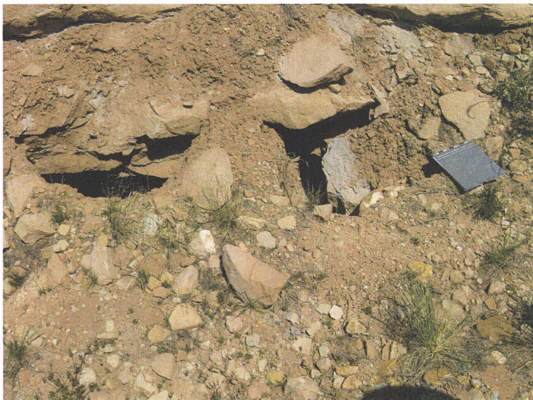
NAD 5/2009. PL-1. Erosion along west side of lower access road (repaired in August 2009).
