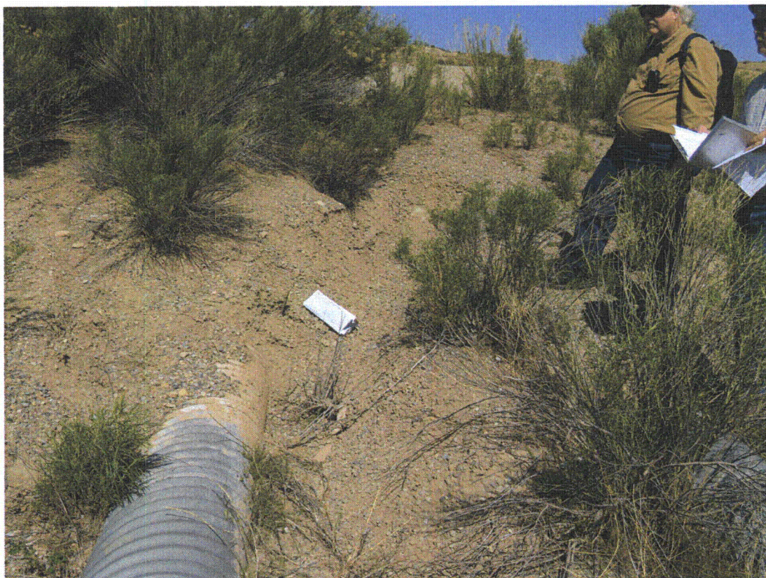
NAD 5/2009. PL-3. View of gullies developing along culverts under the county road.
