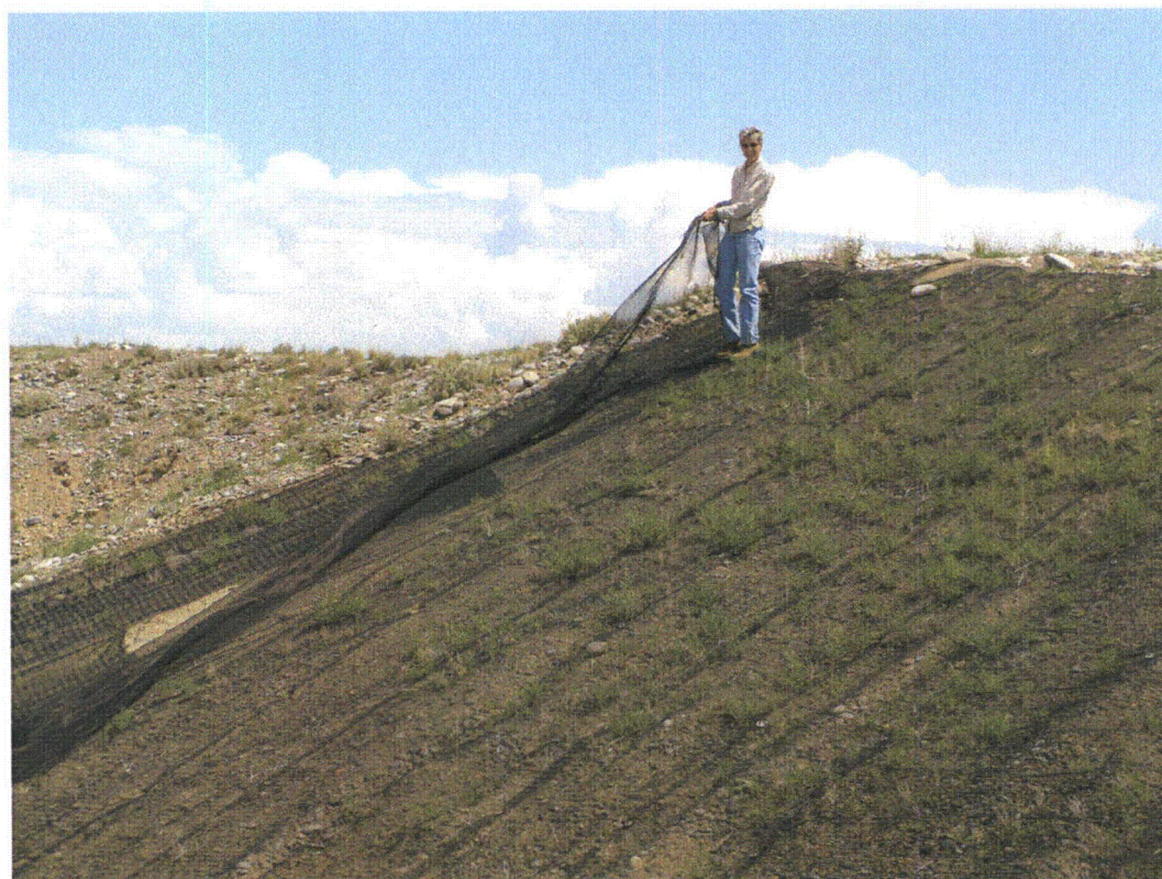
SHP 5/09. PL-4. Loose erosion fabric on the slope of the hill above the outflow channel.
