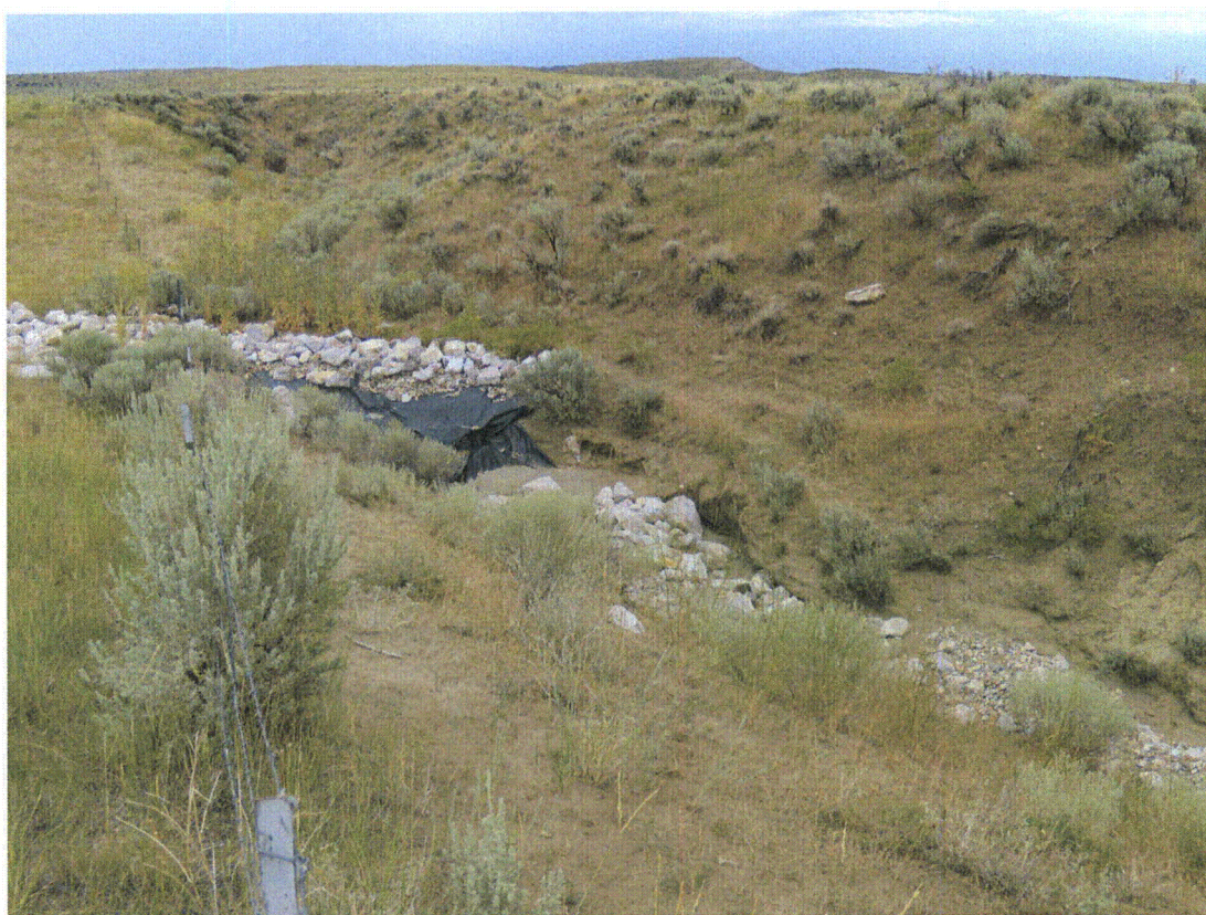
MAY 8/2009. PL-6. Washout riprap at the outlet of Swale No. 1.
