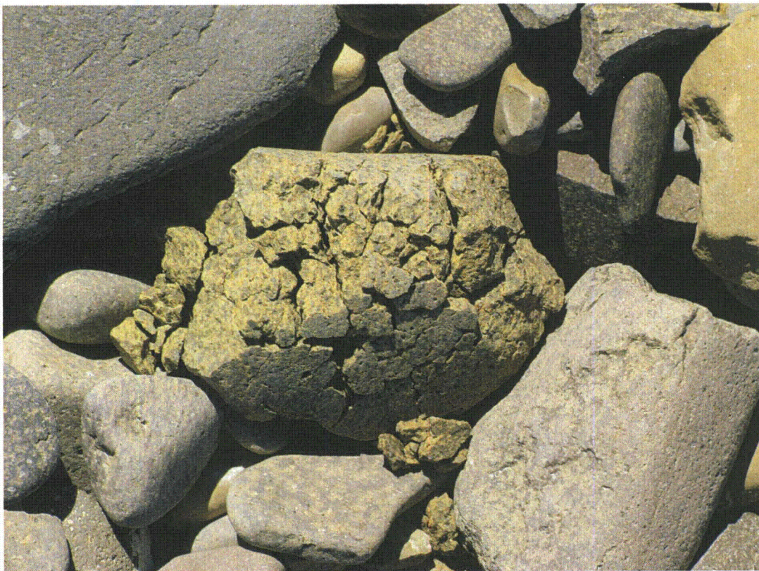
SLC 4/2009. PL-5. Weathering riprap on the disposal cell.
