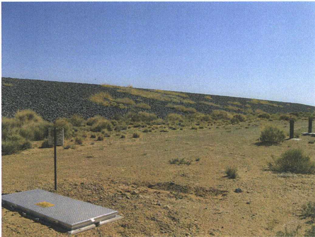
TUB 4/2009. PL-3. Vegetation encroachment on the south side slope of the disposal cell. Photograph taken from extraction well 1107.
