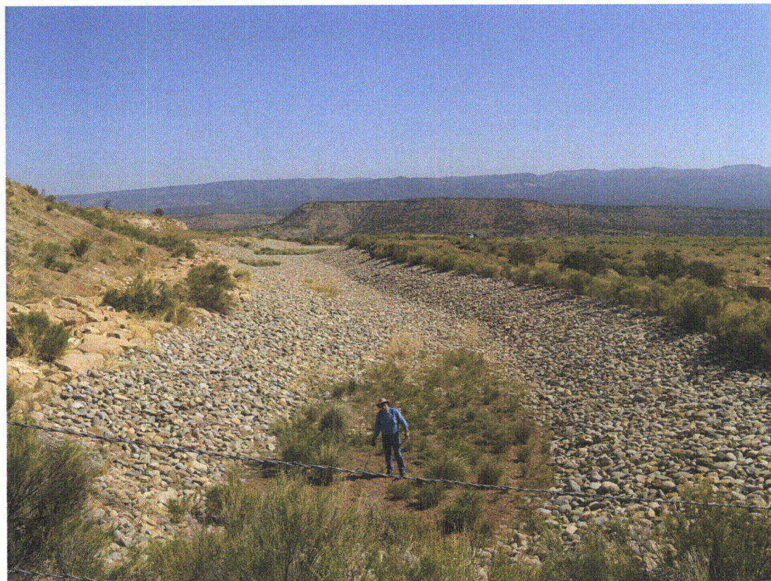
NAD 5/2009. PL-4. Sediment deposition in interceptor channel; small tamarisk/knapweed in center.
