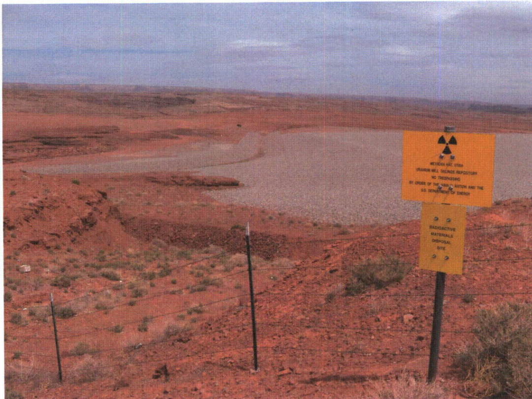
HAT 4/2009. PL-3. West diversion channel and west portion of the disposal cell.
