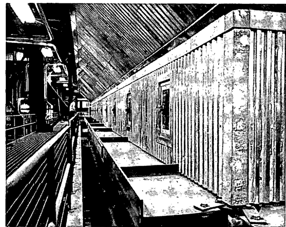
Boiler wall with inspection ports
