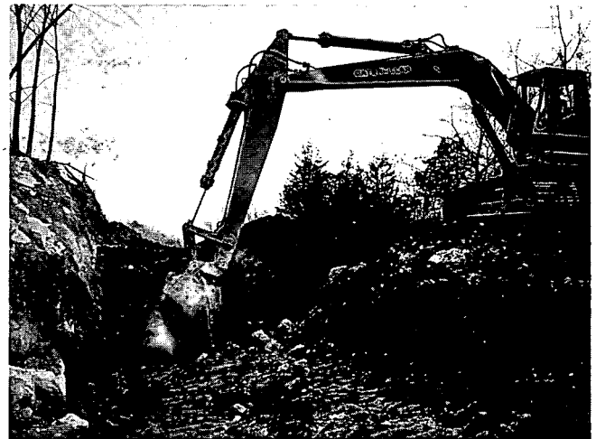
Trenching to uncover bedrock at Cementon
