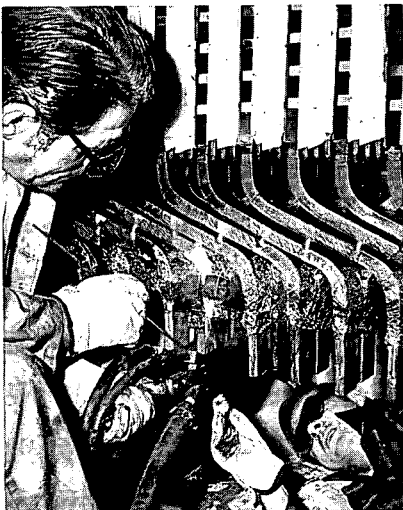
Generator stator rewinding at Niagara
