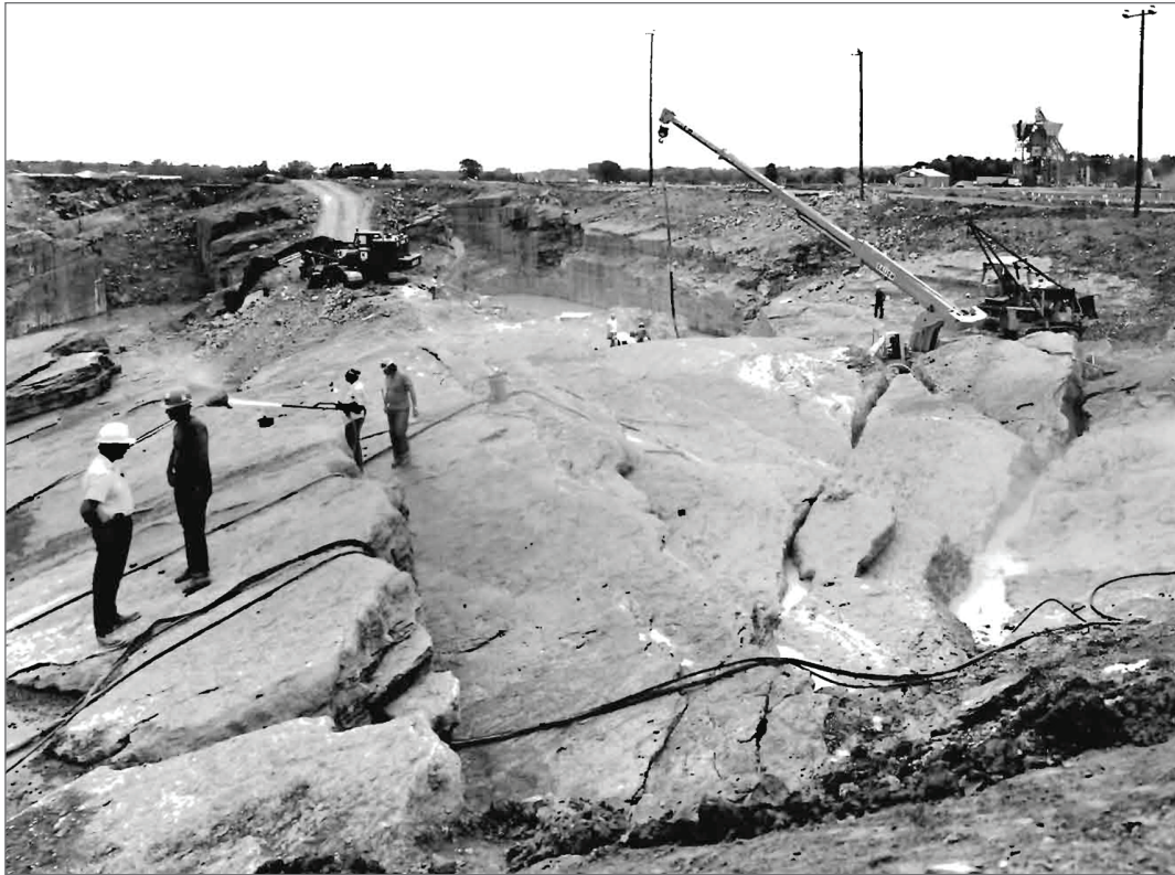
(A) 1975 Excavation for turbine building showing vertical joint oblique to bedding
