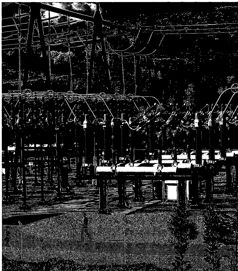
Blenheim-Gilboa's two-way switchyard brings in low-cost electricity to pump water for storage; it also transmits power produced at the project.
