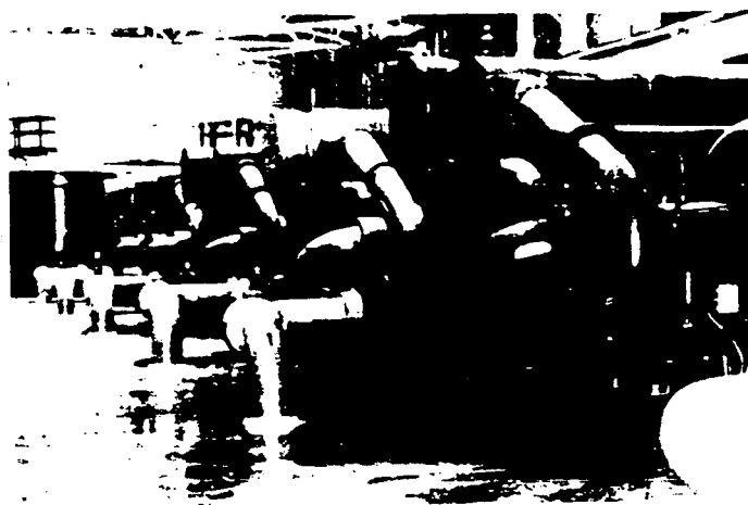
These large pumps are parts of the aqueous-glycol cooling system associated with a major new automobile assembly plant. Courtesy Mogul Corporation
