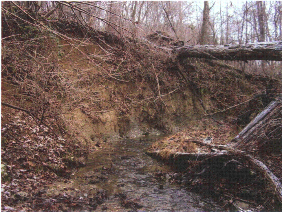
Photo 4-18 Photo depicts a representative section of the proposed mitigation reach along Branch 1. Photo taken looking downstream. Note the 17-foot-high, nearly vertical stream bank (see Concept Plan Sheet 8, Appendix A, SR-3) (November 2008).
