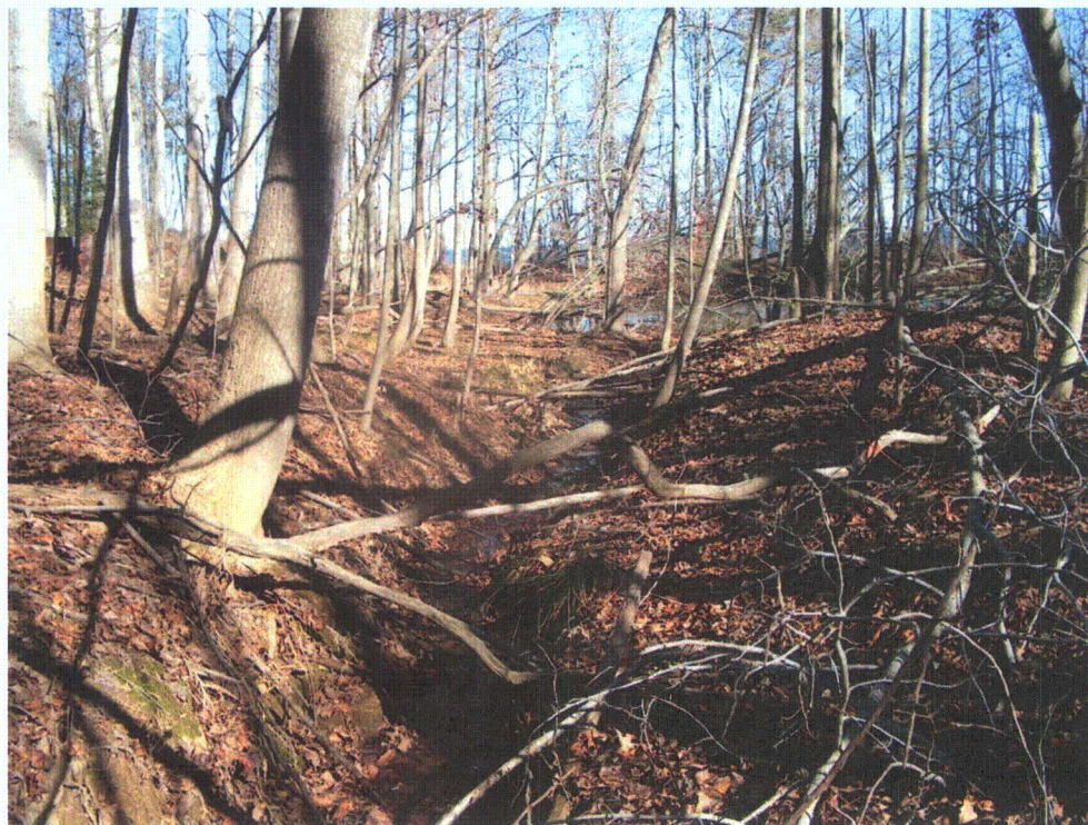
Photo 4-19 Photo of representative section of the proposed mitigation reach along Branch 2. Note the undermined tree roots and small impoundment about 100 feet up stream on this section; photo taken looking upstream. See Concept Plan Sheet 8, Appendix A, SE-4 (November 2008).
