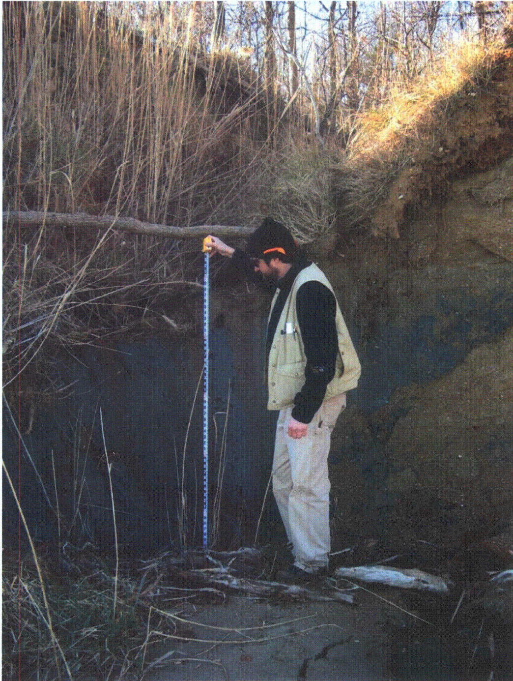
Photo 2-22 Photo depicting the most downstream headcut, located at the confluence to the Chesapeake Bay, the unnamed tributary coming from the historic Camp Conoy Fishing Pond (February 2008).
