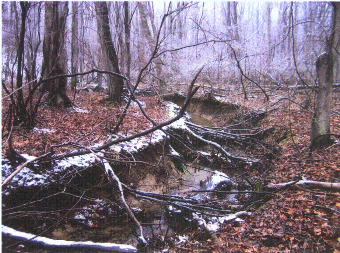
Photo 4-8 Photo depicts a representative section of the proposed mitigation reach along Woodland Branch. Note the roots have been undermined by down-cutting. Photo taken looking upstream (November 2008).
