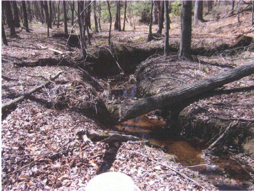
Photo 4-22 Photo depicts a representative section of the proposed mitigation reach along an unnamed tributary to Johns Creek. Note the stream channel is incised in this section. Photo taken looking downstream (November 2008).
