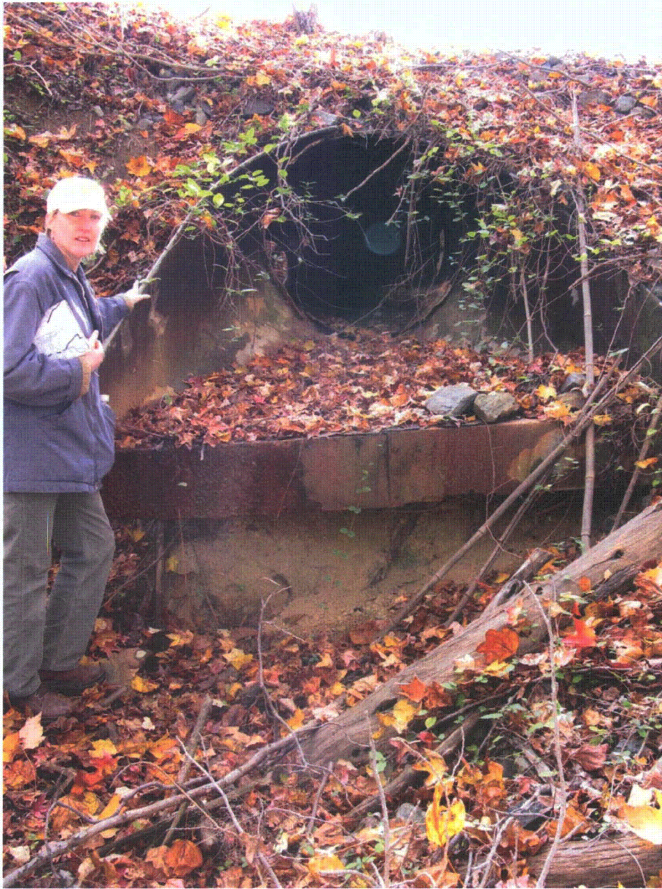
Photo 2-19 Photo depicting a view to the north side, the outlet pipe of the historic Camp Conoy Fishing Pond (November 2008). Photo taken facing south or upstream during high-flow runoff events.
