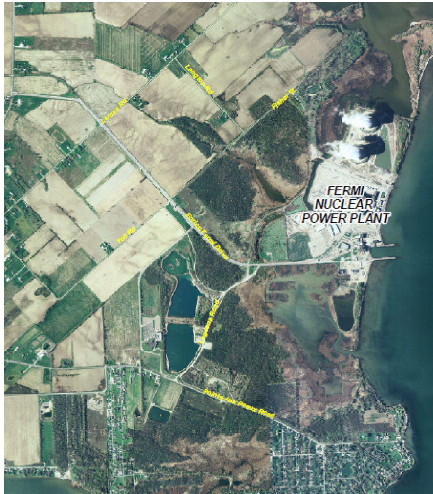
FIGURE 1 Fermi Project Site
