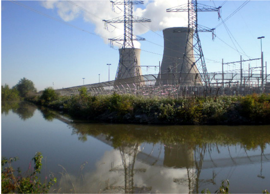
View of northern canal facing northeast
