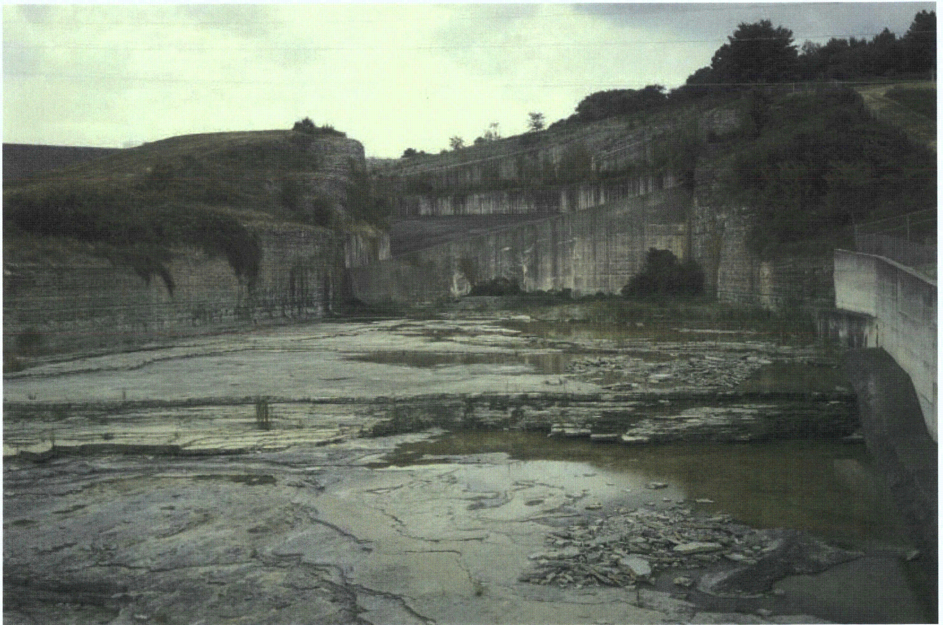
FIGURE 10 - Spillway - Lower End Looking Upstream, July 1999
