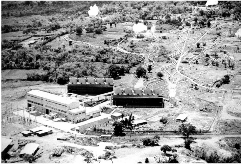
Figure 8.2 Ahuachapan geothermal facility after commissioning around 1977 (DiPippo, 1978).
