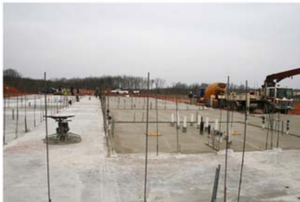
As of February 18, 2009, construction workers have started to pour concrete for the floors of Moss-Nuckols Elementary School.
