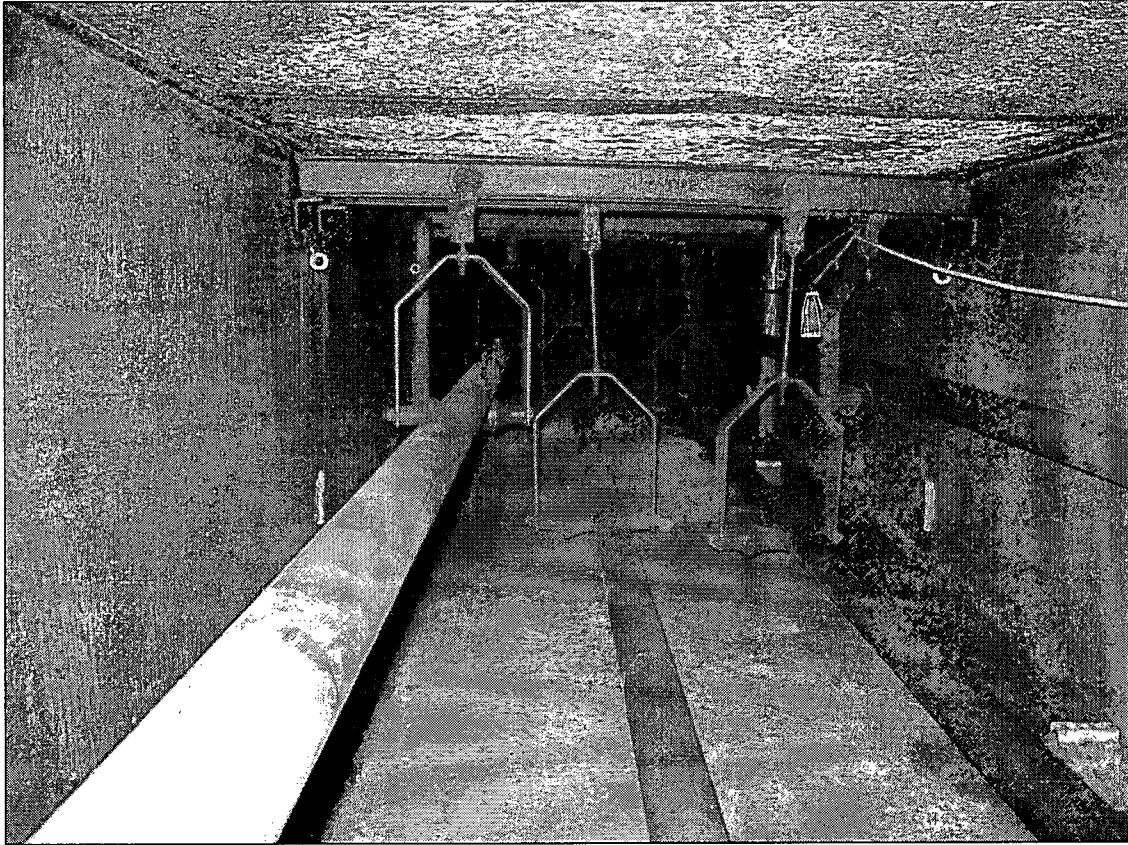
Figure 15 Sodium Tunnel Interior
