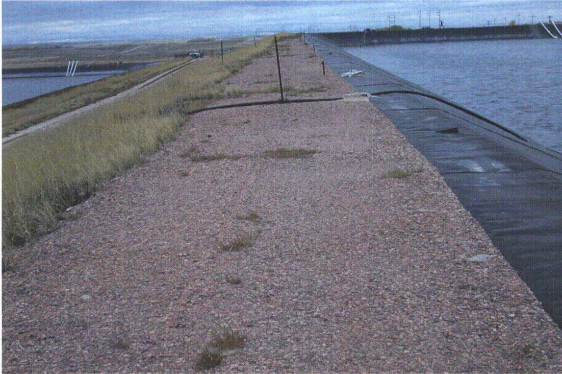
#11 North view of west embankment & berm of pond #1, good protection against erosion of berm & protection of area adjacent to pond liner. 10/20/08
