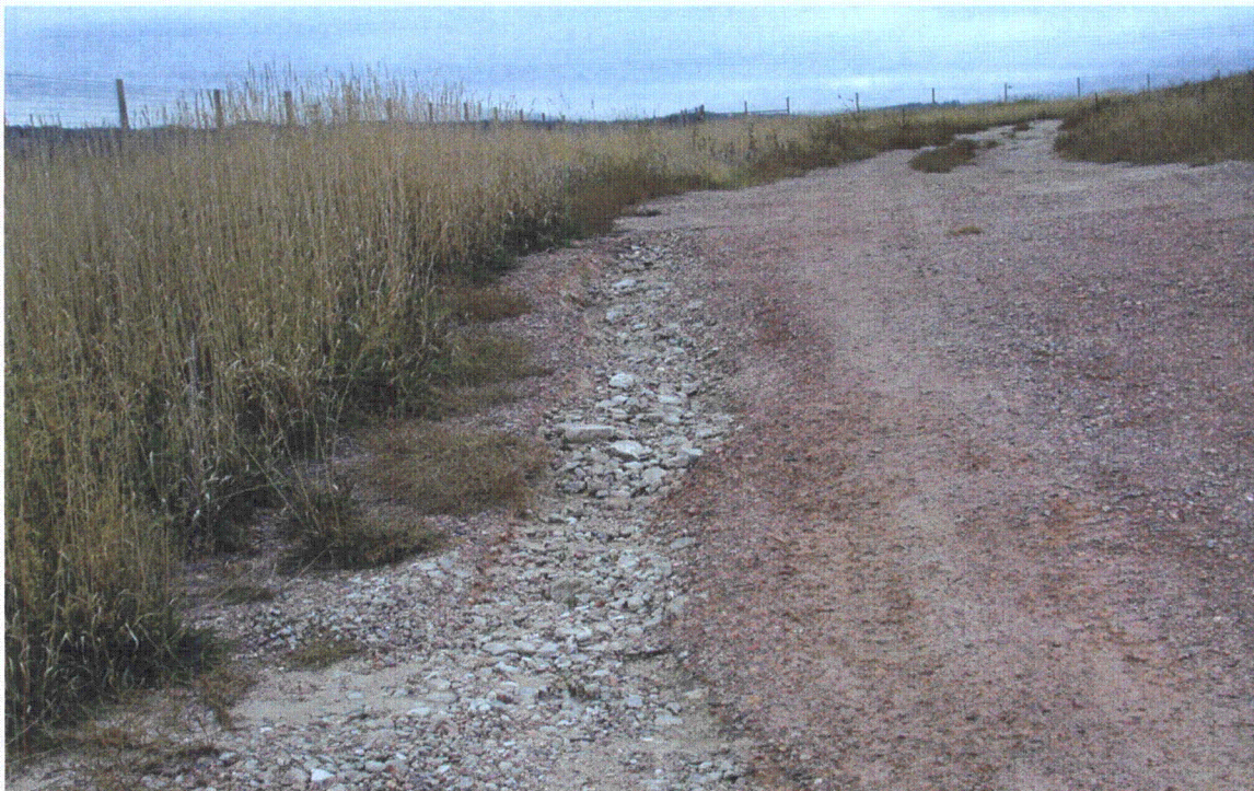
#12 North toe of pond #1 & access road showing erosion ditch on north side. 09/29/09
