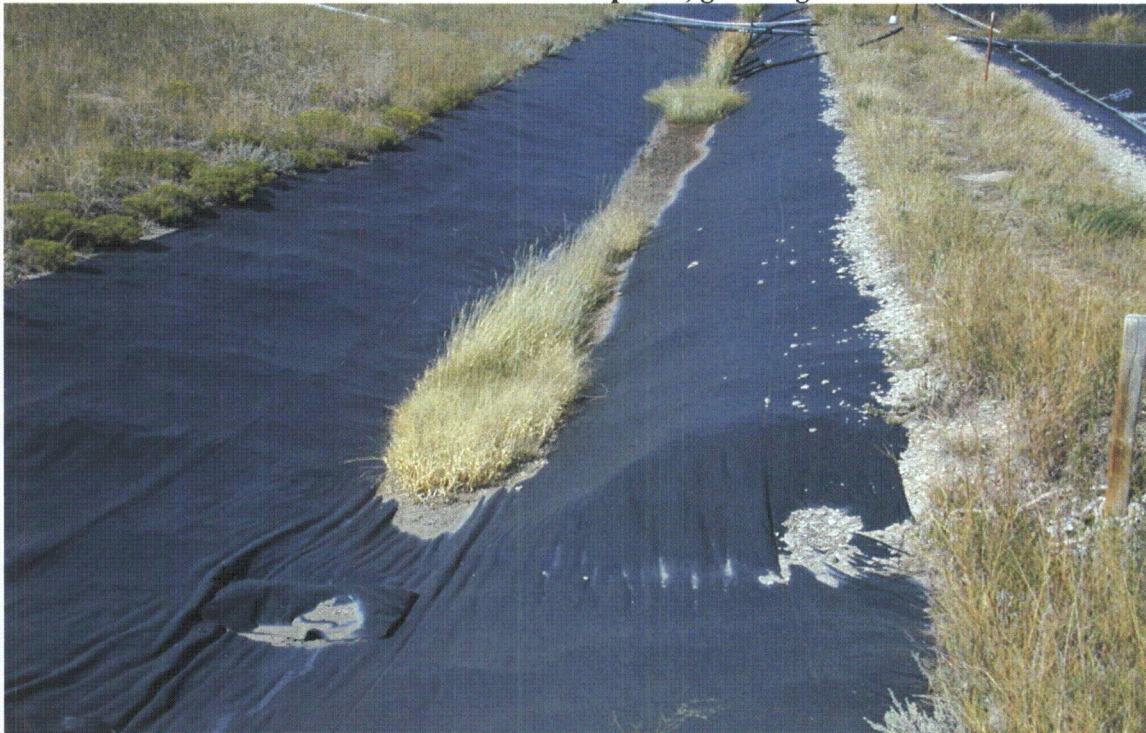
Photo #10 View of diversion ditch on the south side of the R & D ponds Photo taken 09/29/09
