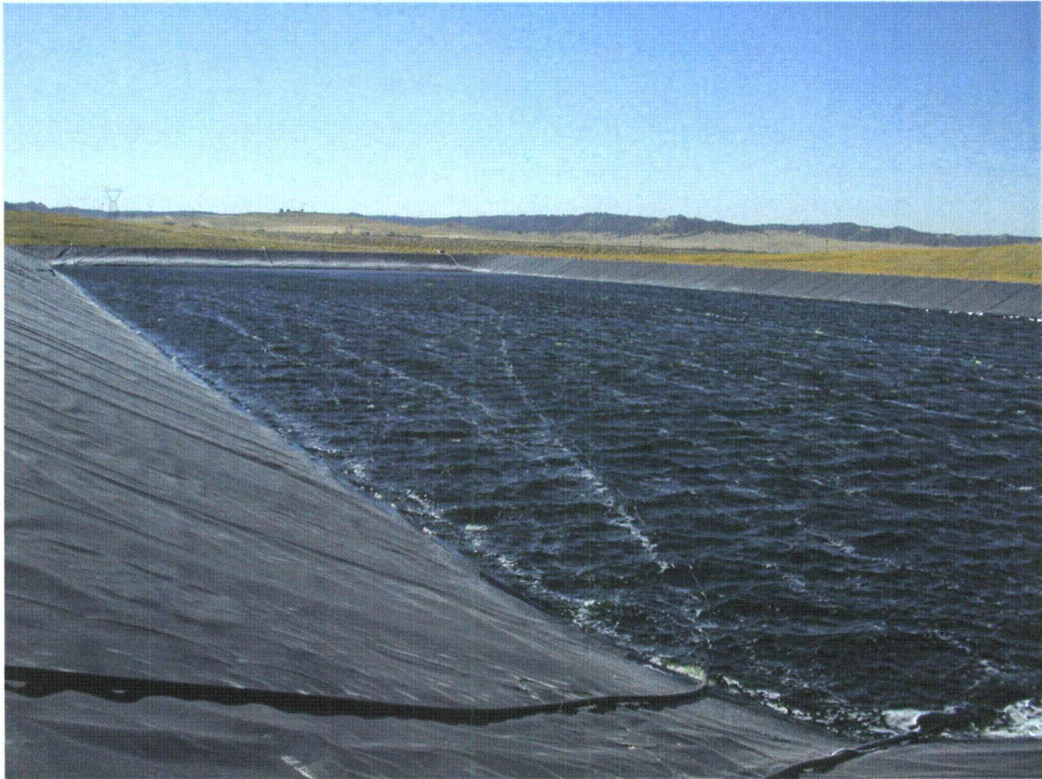
#3 Northeast view of pond #3. Date: 09/29/09
