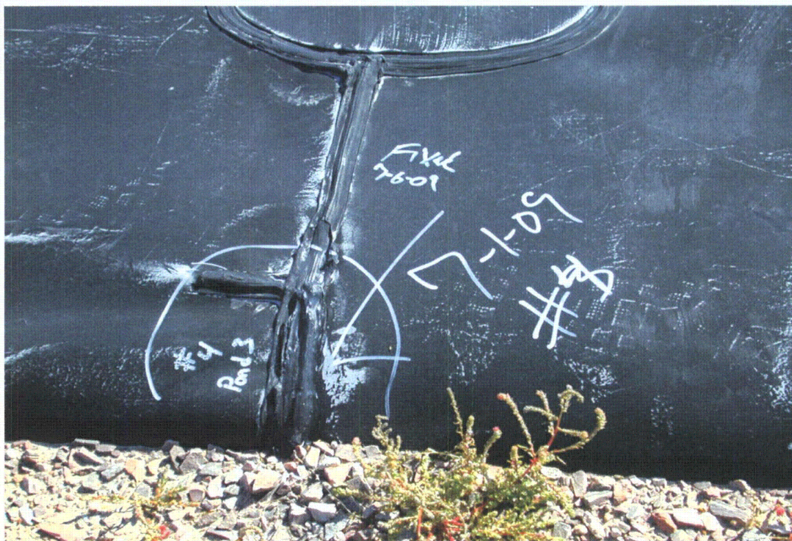
#5 liner repair on Pond #4, Date: 09/29/09
