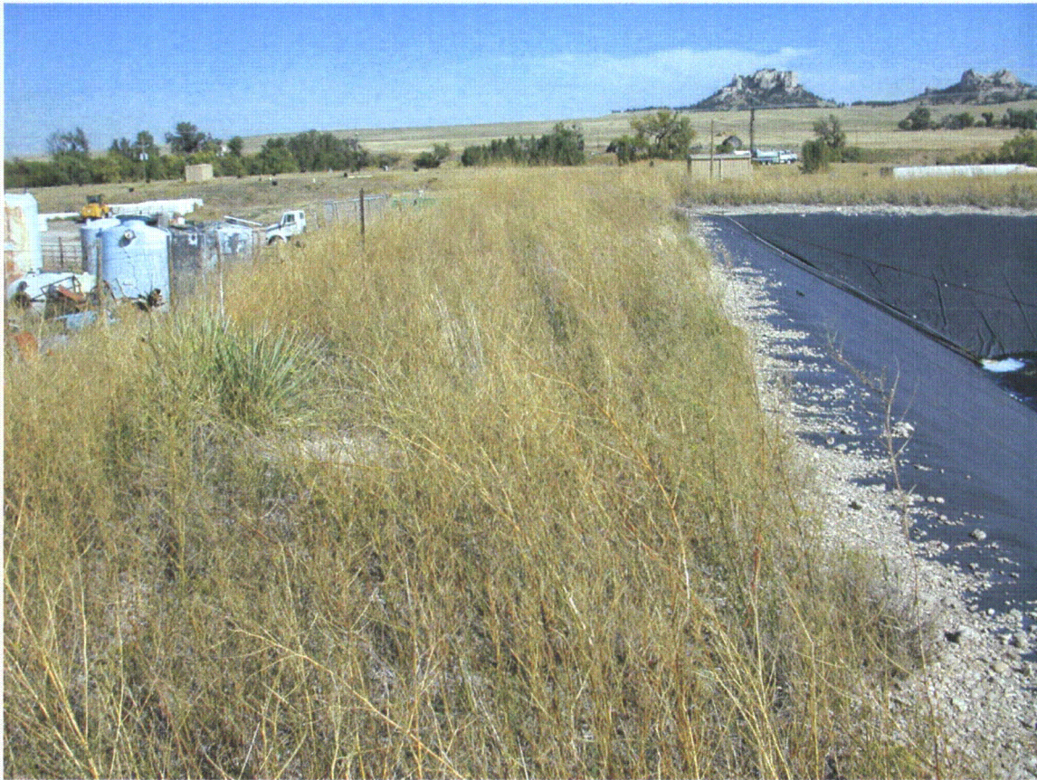
#9 West view of south embankment of R & D ponds, good vegetation: Date: 09/29/09
