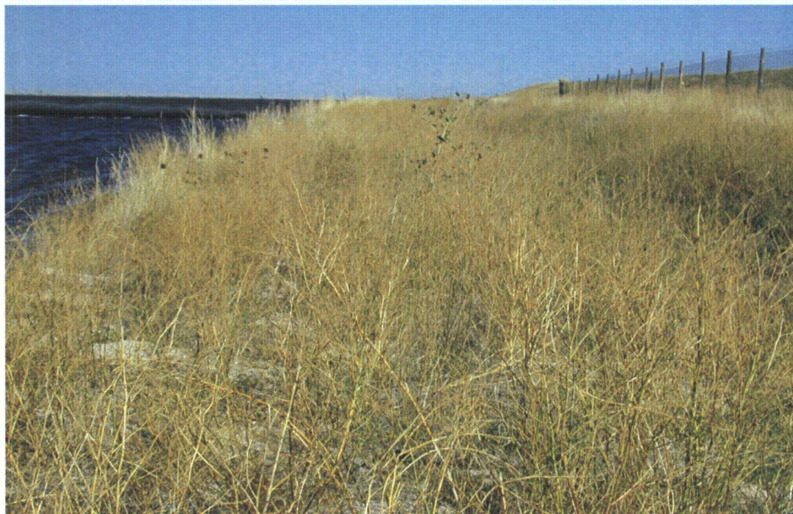
#6 View of vegetation & toe of slope of pond #4, looking to the north. Date: 09/29/09
