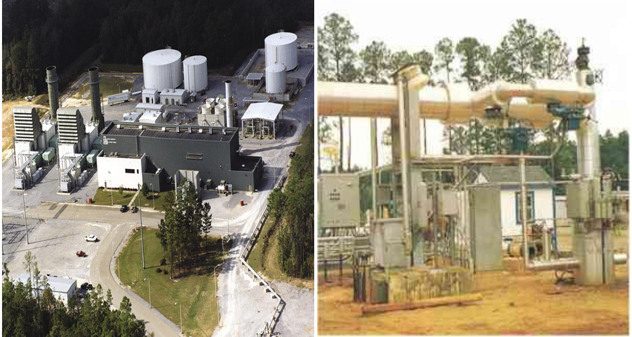
Figure 3. The Alabama Electric Cooperatives' McIntosh, Alabama 110-MW CAES power plant with compressed air well-head on the right. The power plant has been in continuous operation since 1991.
