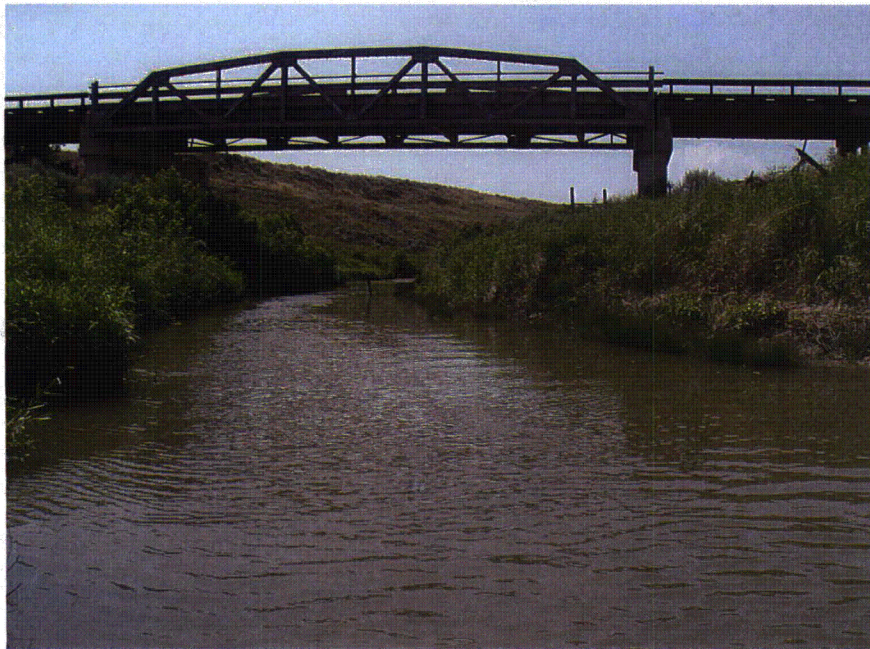
Photo 45. Site BVC04 looking upstream from Transect 10 July 8, 2008.
