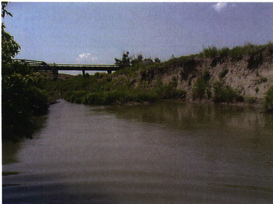
Photo 41. Site BVC04 looking upstream from Transect 6 July 8, 2008.
