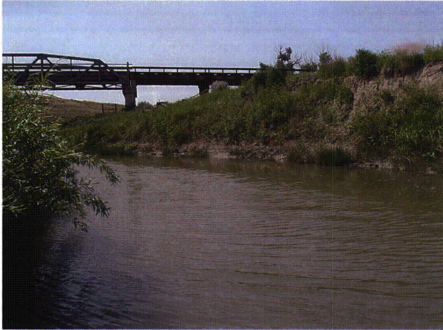
Photo 44. Site BVC04 looking upstream from Transect 9 July 8, 2008.
