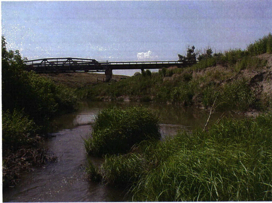
Photo 42. Site BVC04 looking upstream from Transect 7 July 8, 2008.
