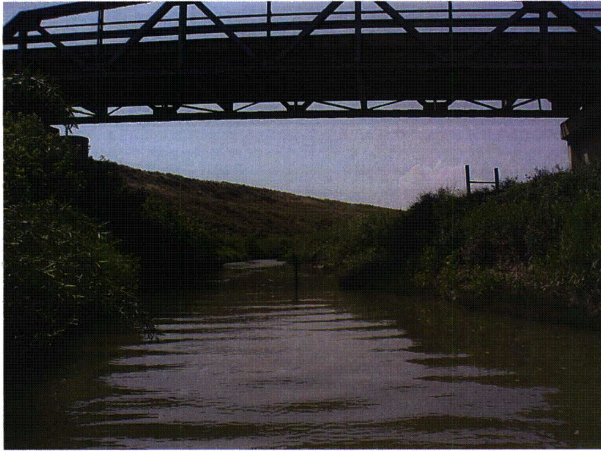
Photo 46. Site BVC04 looking upstream from Transect 11 July 8, 2008.
