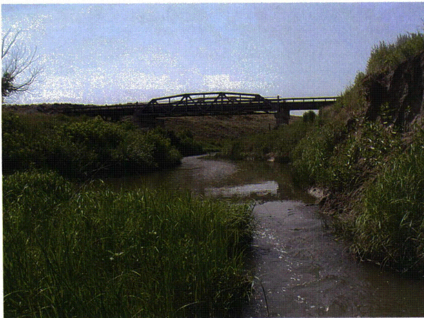
Photo 43. Site BVC04 looking upstream from Transect 8 July 8, 2008.
