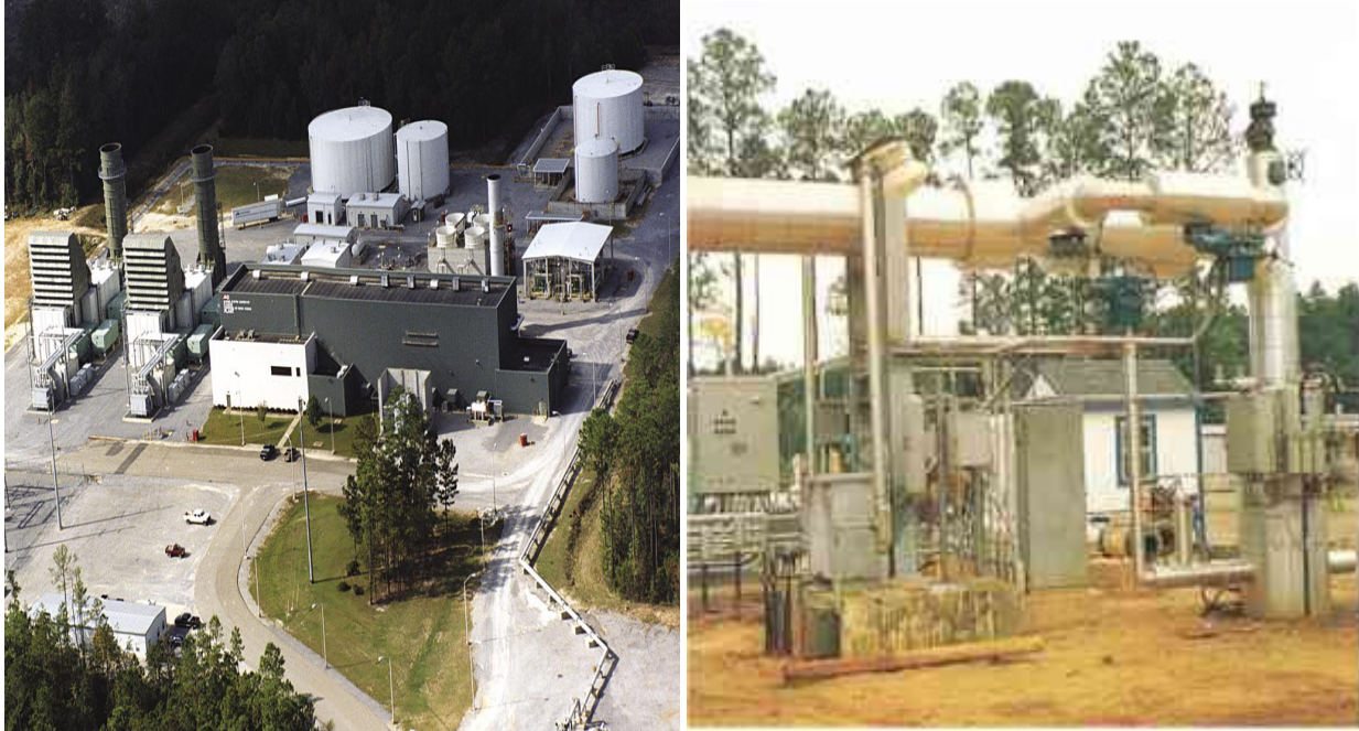
Figure 3. The Alabama Electric Cooperatives' McIntosh, Alabama 110-MW CAES power plant with compressed air well-head on the right. The power plant has been in continuous operation since 1991.
