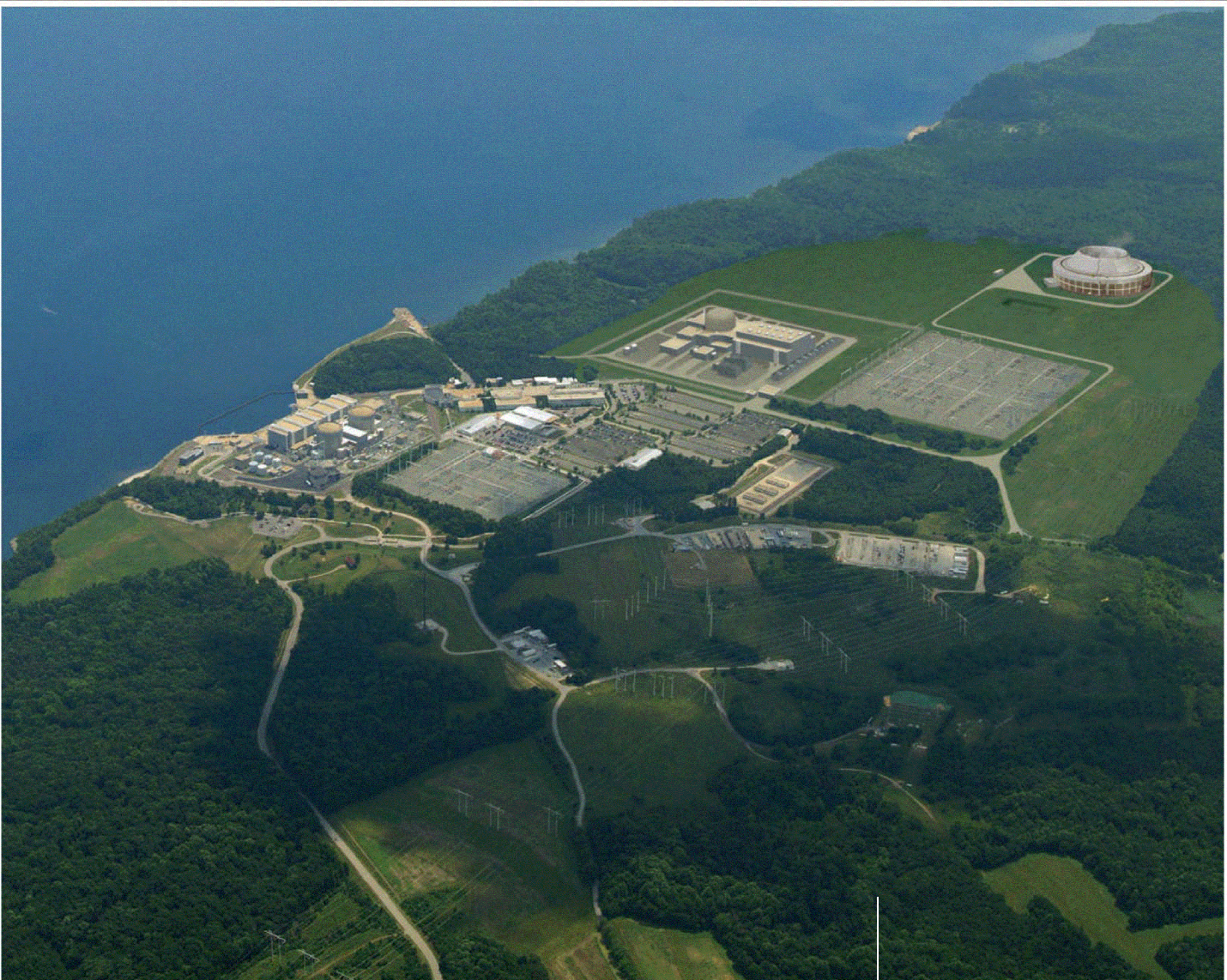
Figure 1.2-4—Aerial View of CCNPP Units 1 and 2 with CCNPP Unit 3 Superimposed
