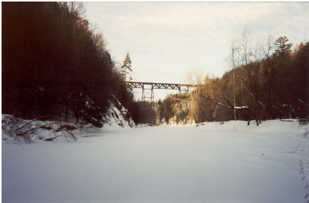
Figure 10. The bridge over Cattaraugus Creek, used to transport materials into and out of West Valley until 1998, was originally built in 1898. 59
