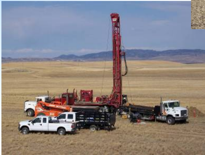
Monitor Well Installation at the Shirley Basin South, WY, Disposal Site
