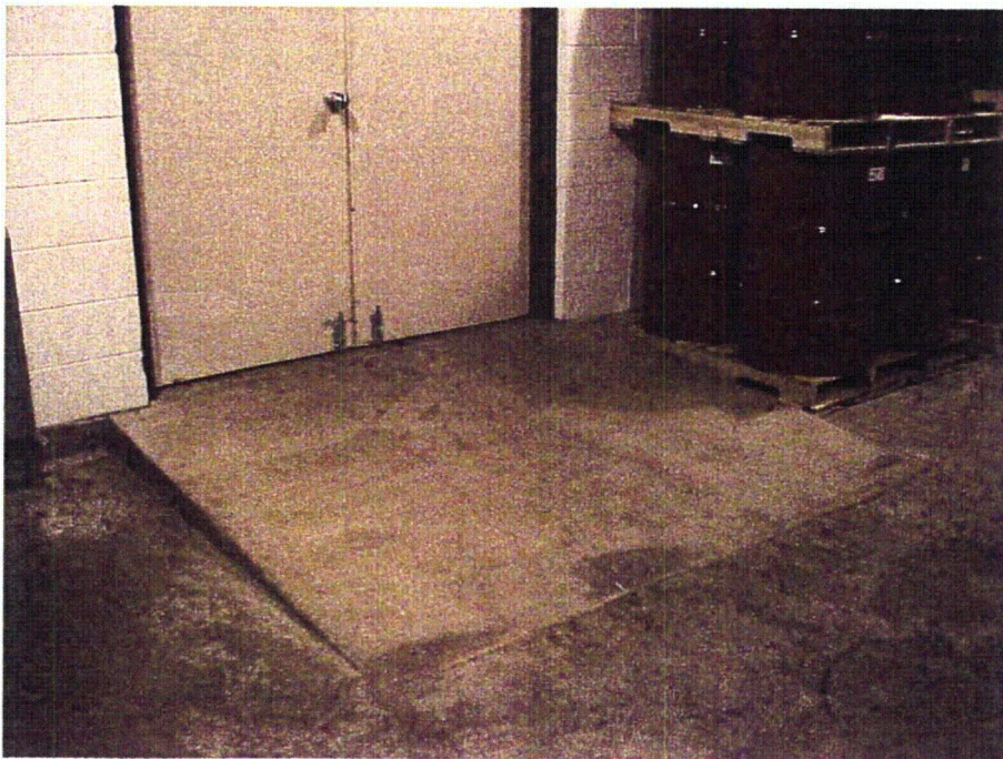
Photo 34: Office/Warehouse Annex Drum Storage; Used Oil. Entrance door has ramp that acts as containment berm.
