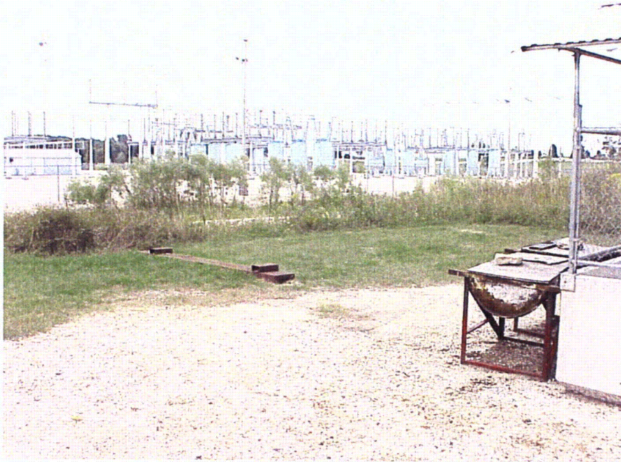
Photo 31: ATC/Dominion Switchyard area in the background.
