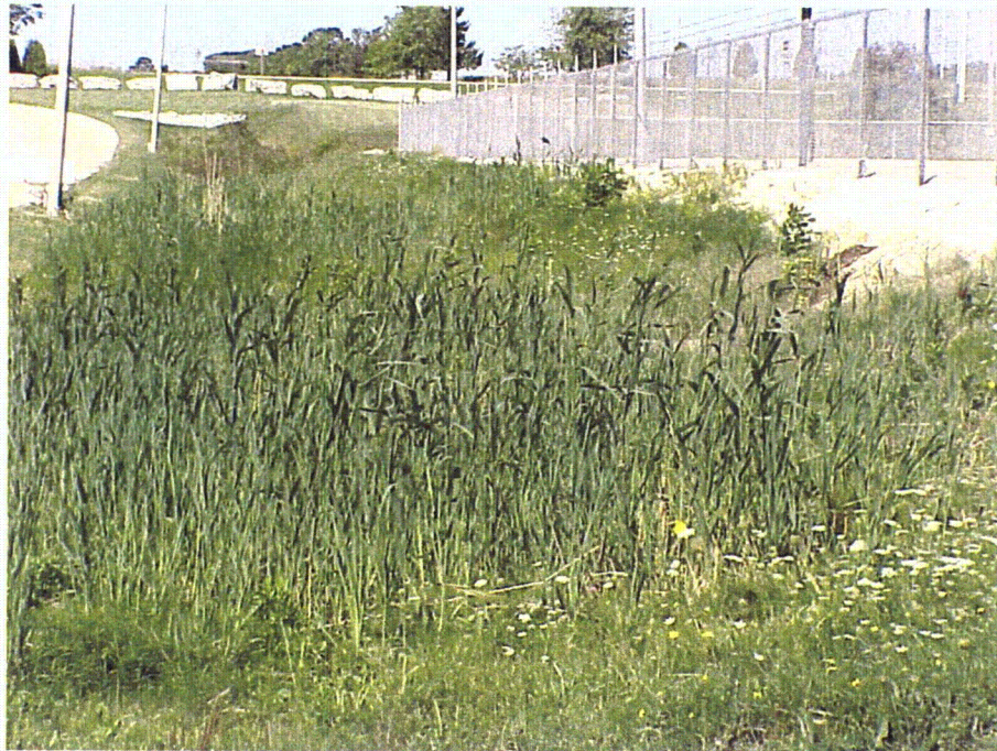
Photo 52: Flow Route of Runoff from Transformer Switchyard.
