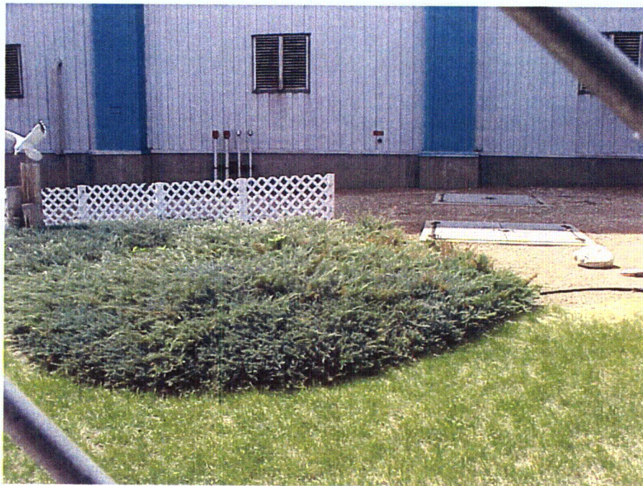
Photo 12: Photo of the area where the 35,000 gallon USTs are located.
