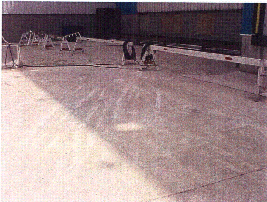
Photo 22: 30,000 Gallon Boiler Fuel Oil Tank Truck Unloading Area is in Vicinity of Lake Michigan Stormwater Drainage Grate.
