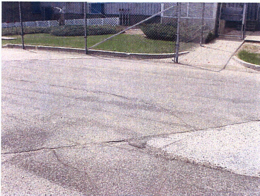
Photo 14: Photo of the truck unloading area for the 35,000 gallon USTs.
