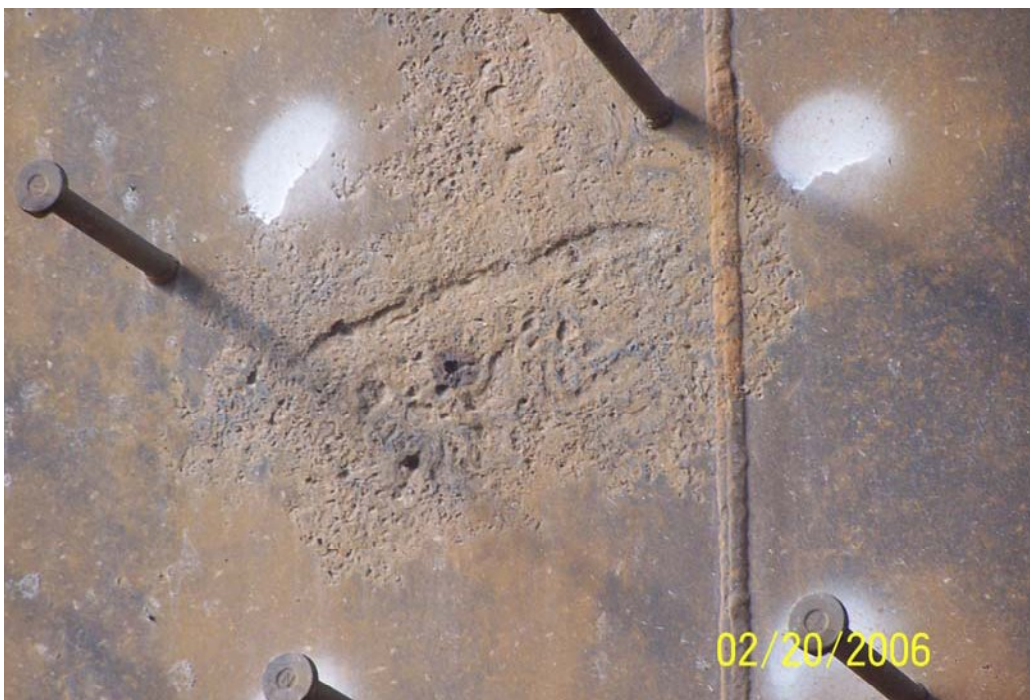
Figure 6: Area 2, Degradation within the BV-1 Containment Construction Opening
