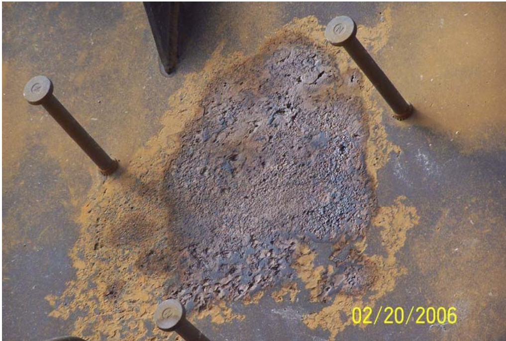
Figure 5: Area 1, Degradation within the BV-1 Containment Construction Opening
