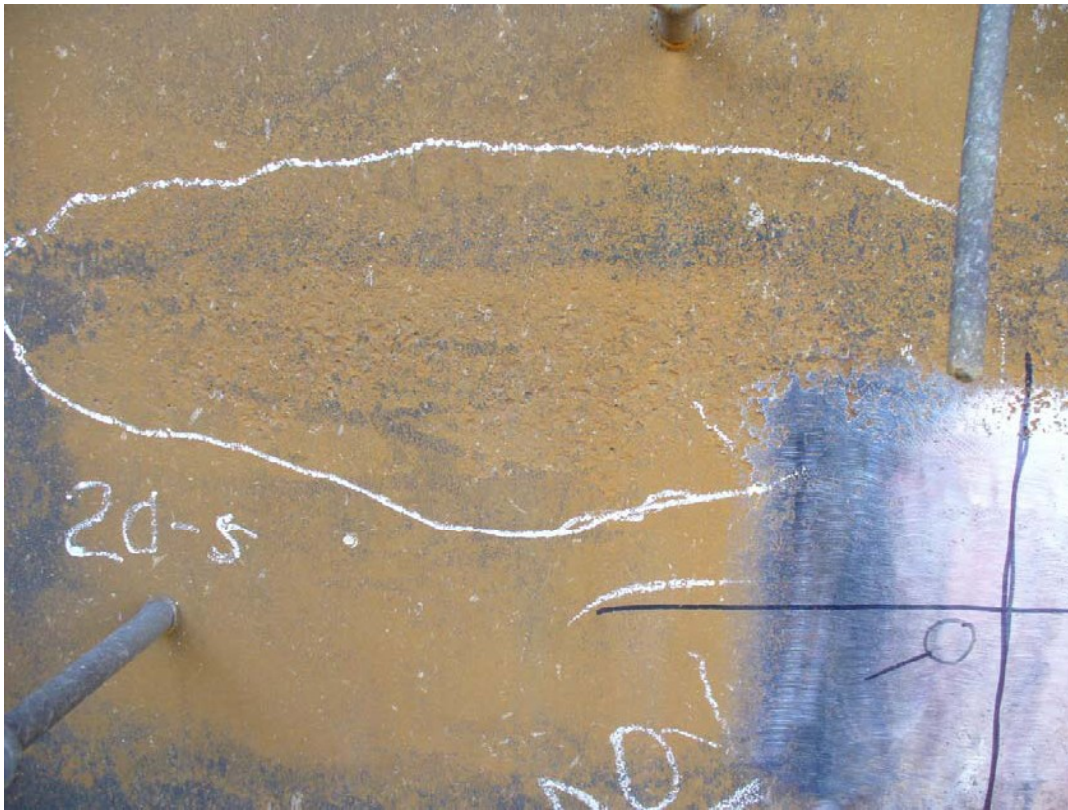
Figure 7: Area 3, Oval of General Near Surface Corrosion within the BV-1 Containment Construction Opening
