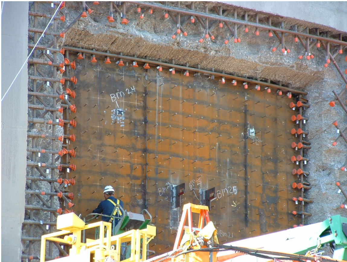
Figure 3: Containment Construction Opening at Another Site
