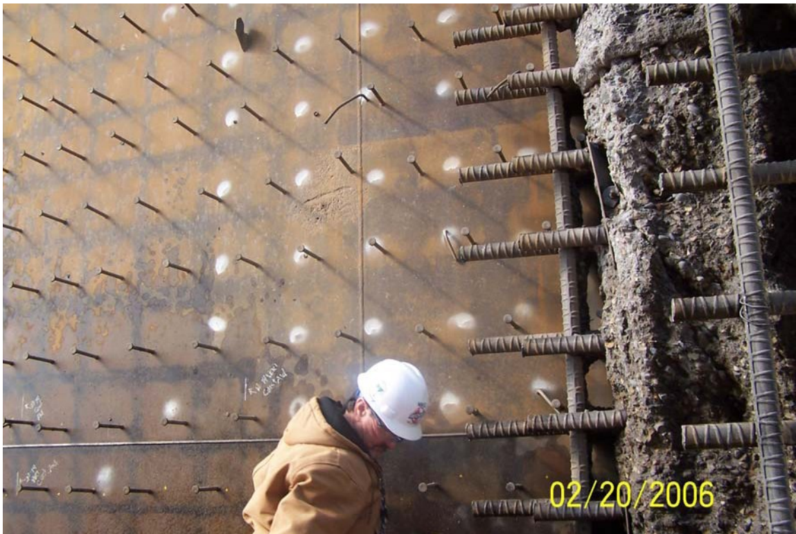
Figure 1: BV-1 Containment Construction Opening (Area 2)
