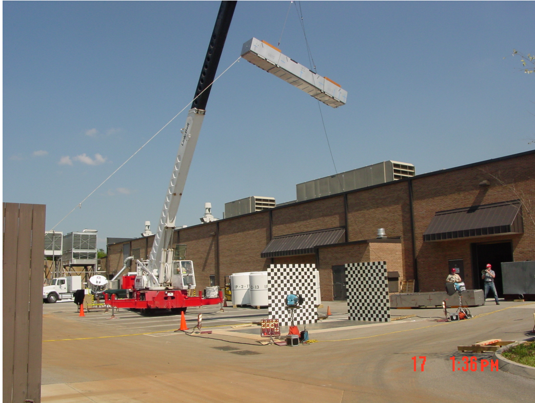
Figure 2-25 CTU 1 Positioned for 15° 9-m (30-foot) Slap-down Drop
