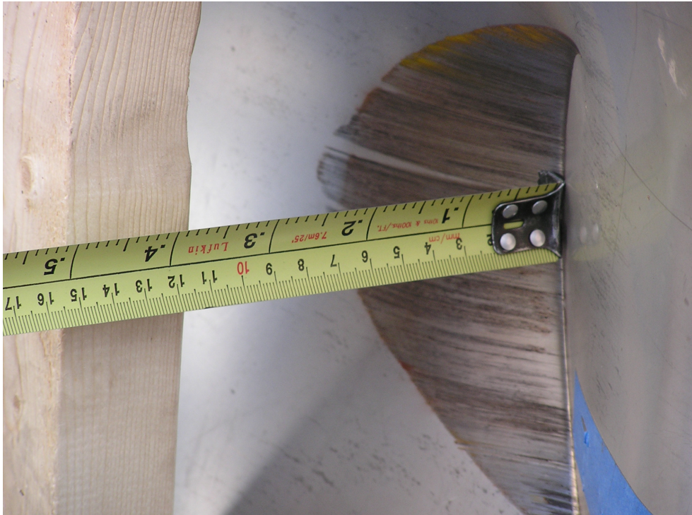
Figure 2-32 Close Up of Puncture Damage
