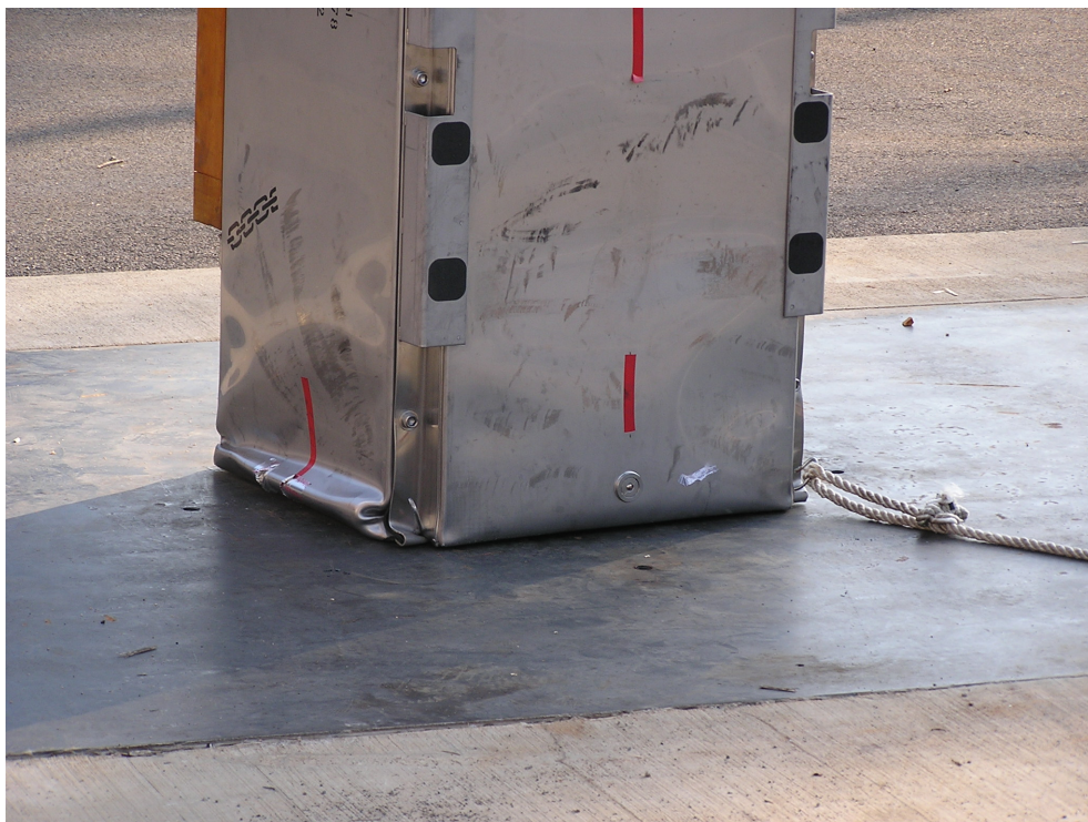
Figure 2-35 End Impact Damage (Top and Side)
