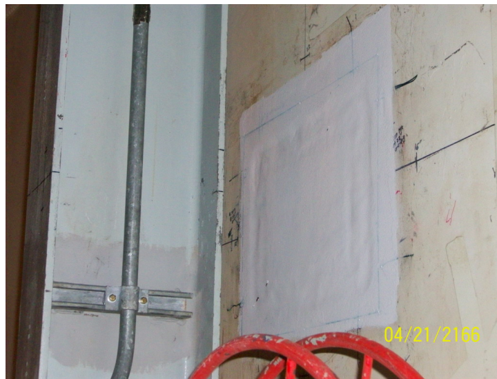
BEAVER VALLEY UNIT 1 LINER REPAIR
