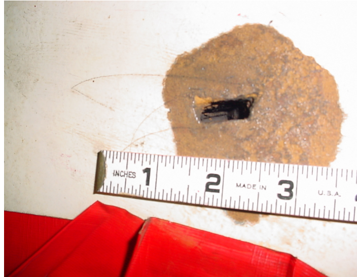
BEAVER VALLEY UNIT 1 LINER HOLE
