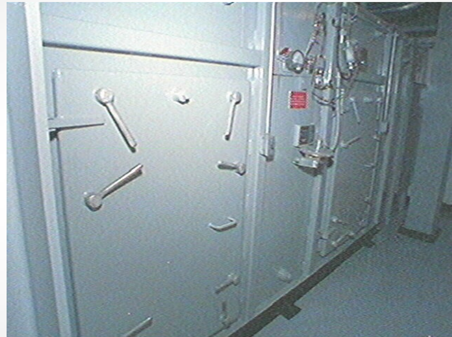
Auxiliary Building Filter 1-HV-FL-3B
