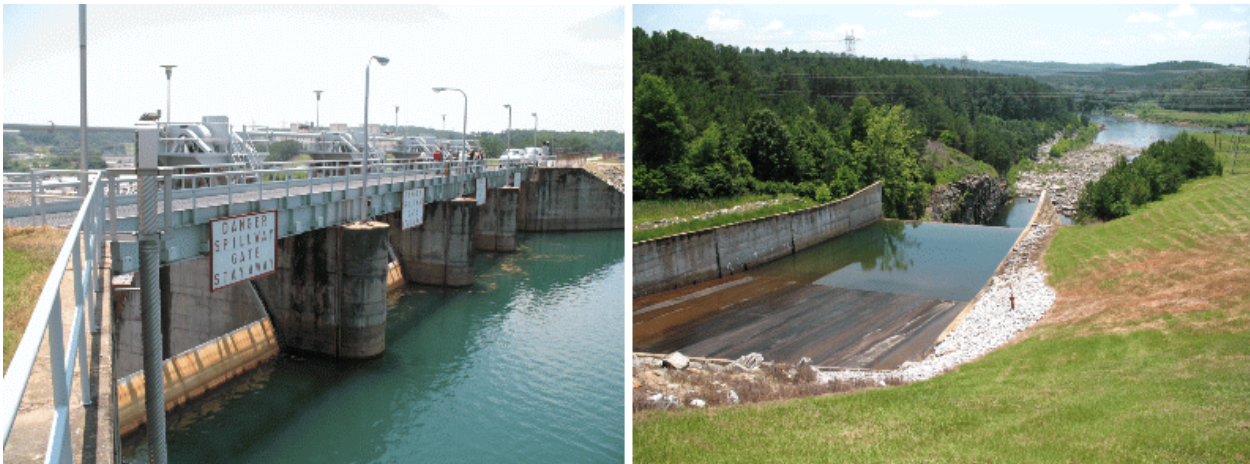
Keowee Dam spillway with four radial gates (left), and view of outflow channel (right).
