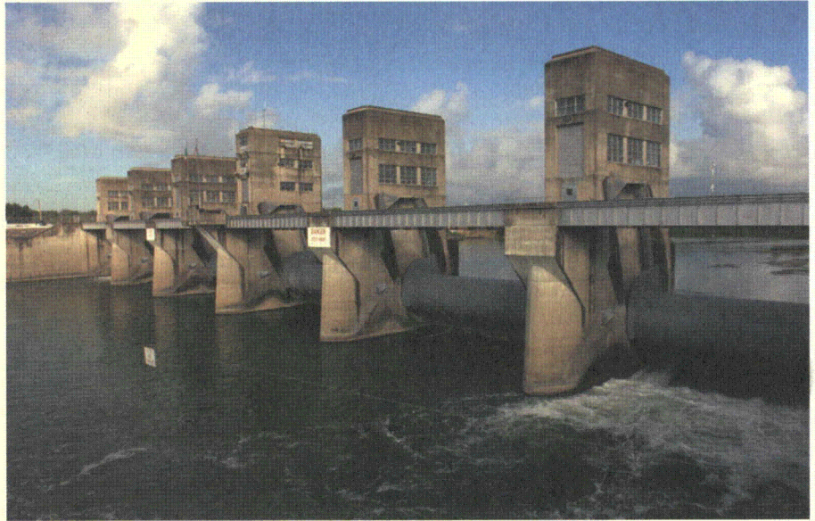
Anzalduas Dam, TX. Photo courtesy International Boundary & Water Commission.
