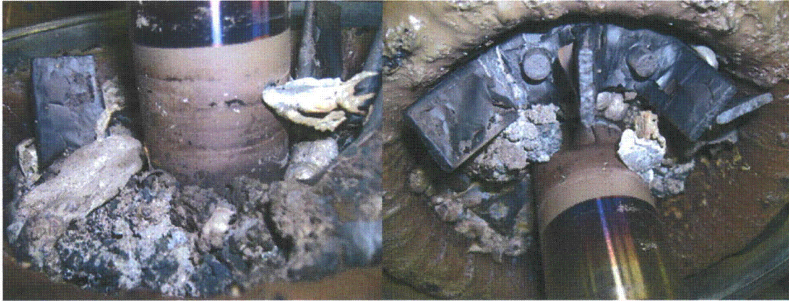
Figure 9 - Catastrophic failure of magnesium rotor where the magnesium casting melted during a locked rotor condition.
