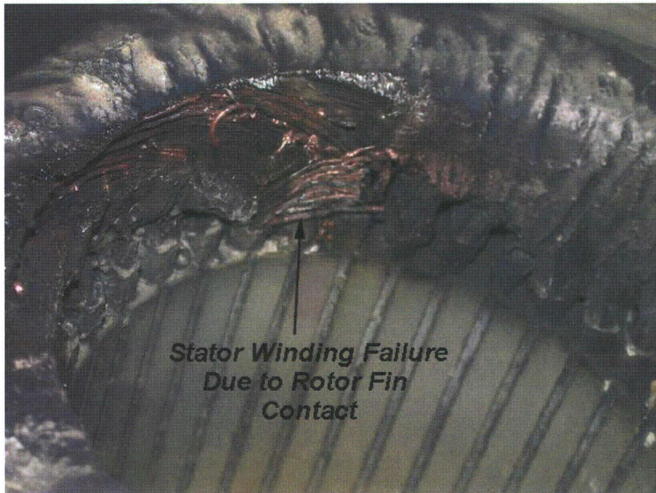
Figure 8 - Motor stator winding failure due to motor rotor cooling fins contacting the stator winding during operation. The cooling fins were deflected due to corrosion products between the end lamination and magnesium end ring.
