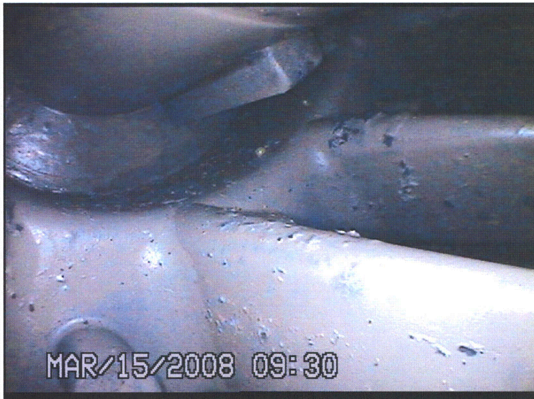
Figure 34 – Slight blistering onset of corrosion of the magnesium end ring/cooling fins coating.
