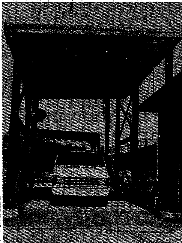
Fig. 19.12 The components of this vehicle monitor carry out the same basic functions as a pedestrian monitor. (Manufactured by Jomar Systems, Inc., Los Alamos, New Mexico.)
