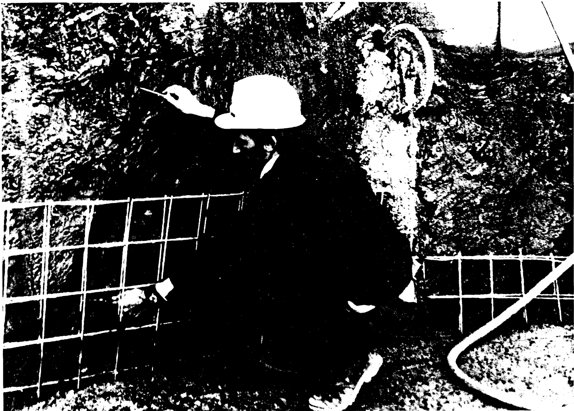
Watts Bar Nuclear Plant Tennessee Valley Authority 90863 P February 20, 1974 Gary W. Krantz, Knoxville Fault in Reactor #2 Cavity Wall at approximately 354 degrees. Elevation 680.0 at base. Viewed southwest.
